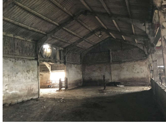
Fig 06. Internal view looking east
