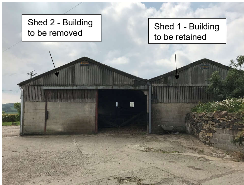
Fig 10. View of gable wall of single storey buildings looking south.
