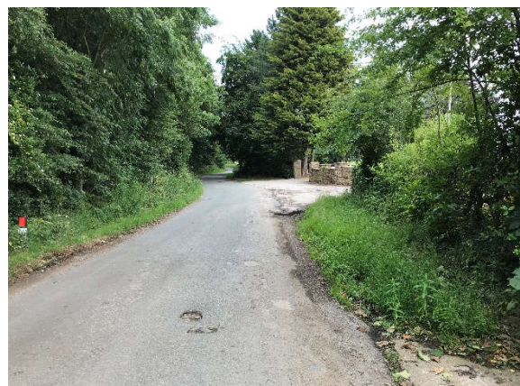
Fig 13. View from access looking n-east.
