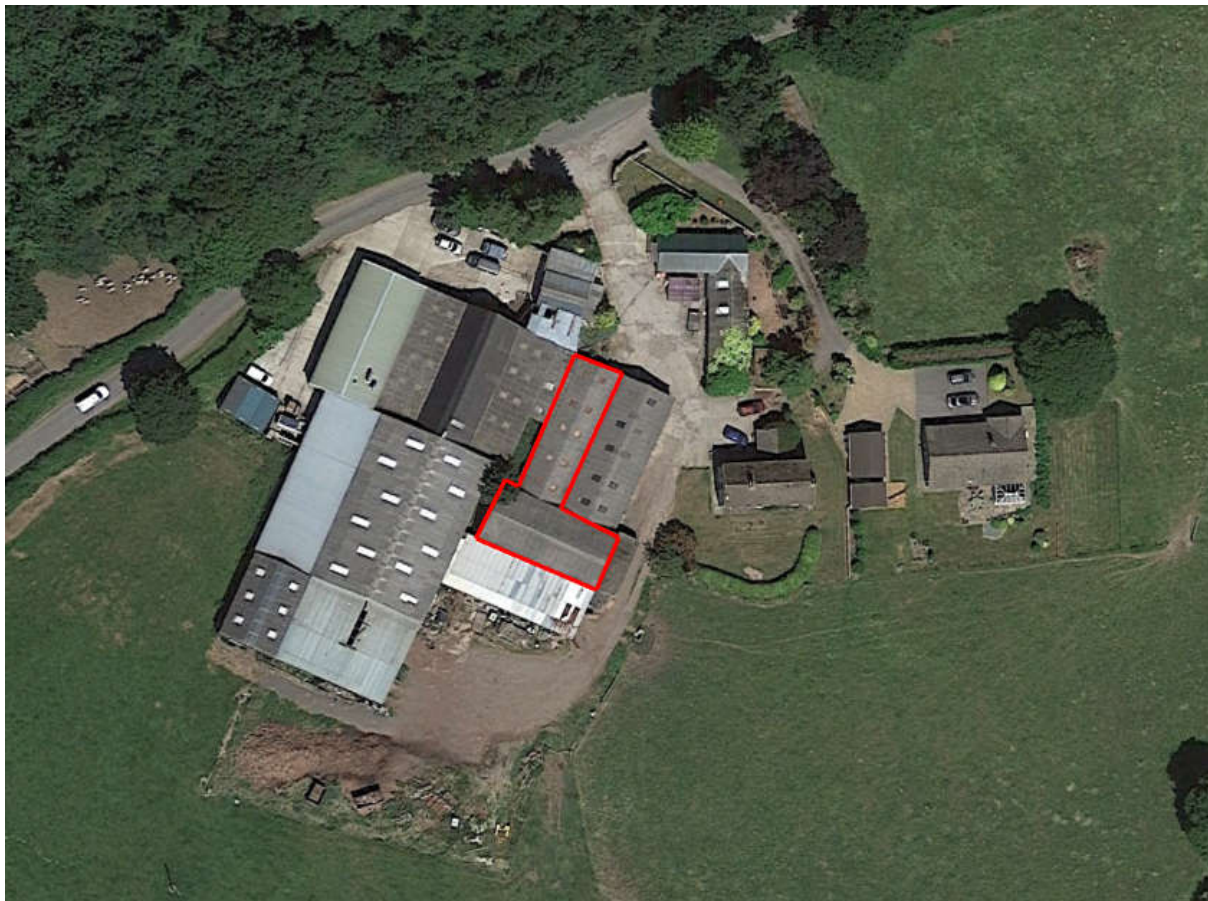
Fig 01. Aerial View of the site showing the proposed change of use buildings edged in red.
