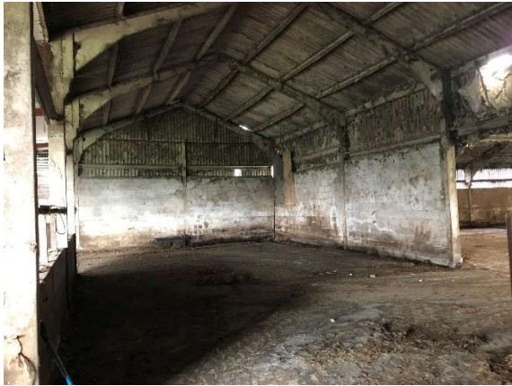
Fig 05. Internal view looking west.
