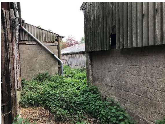
Fig 07. Narrow view of west elevation.
