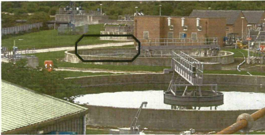
ASP MCC Kiosk Location
