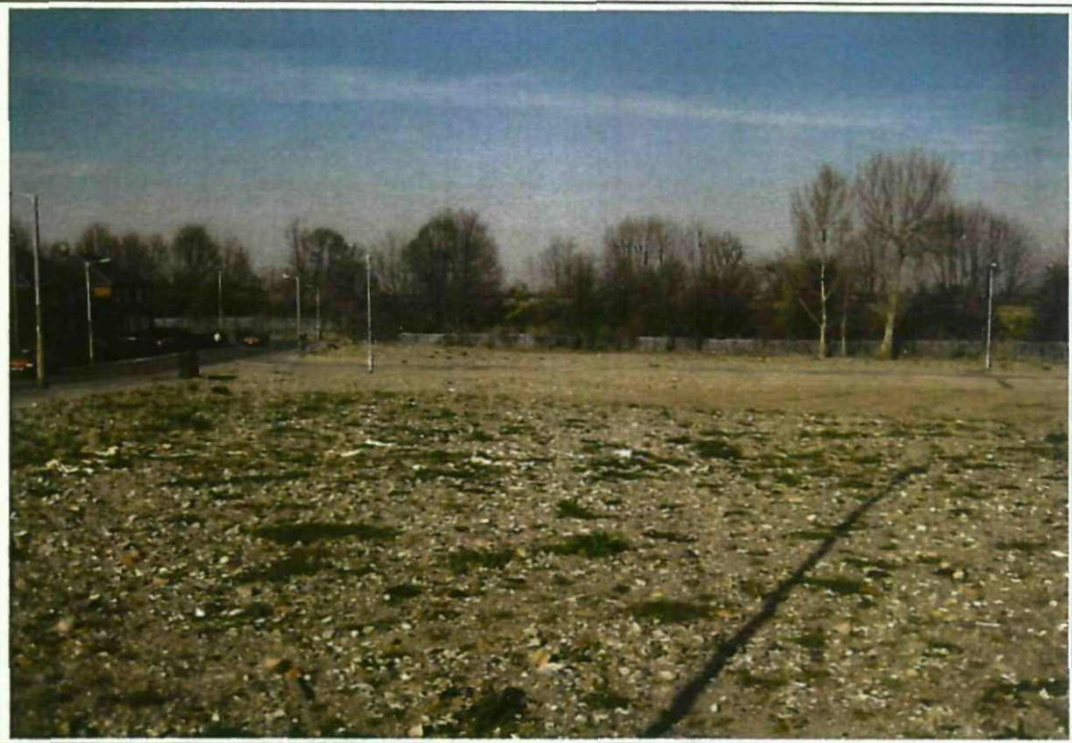
PHOTOGRAPH 3-Low spot against rail embankment in NE corner
