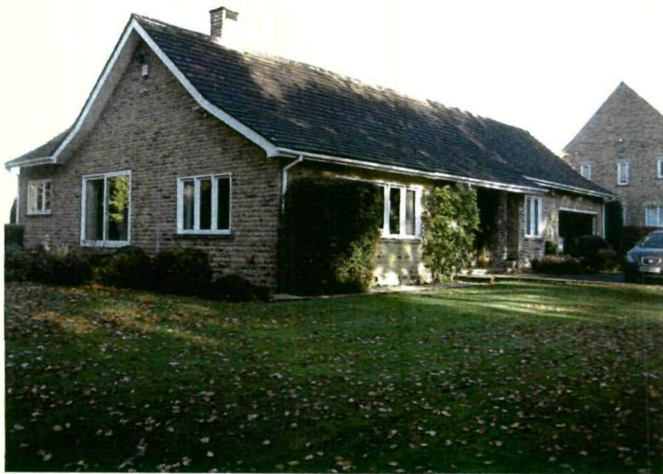
5. Front and side view from the south west
