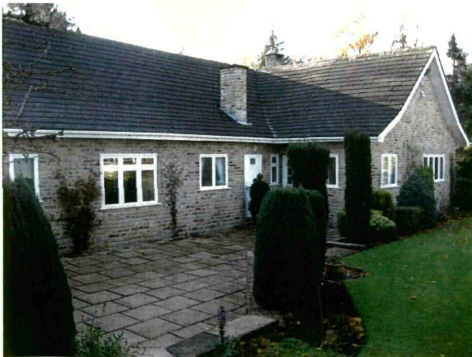
2. Rear elevation viewed from the north east
