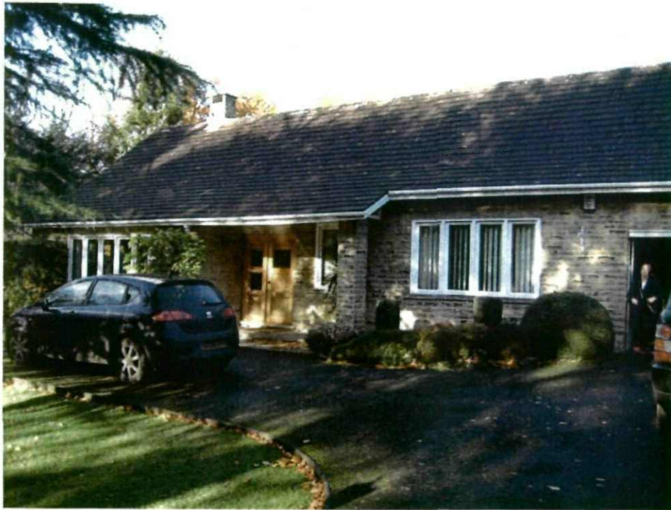
1. Front elevation viewed from the south east
