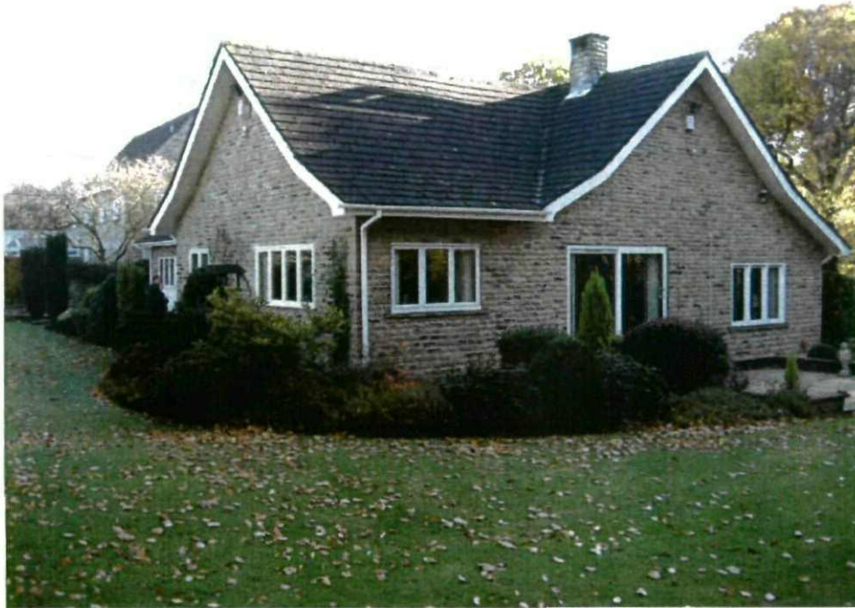
3. Side and rear view from the north west
