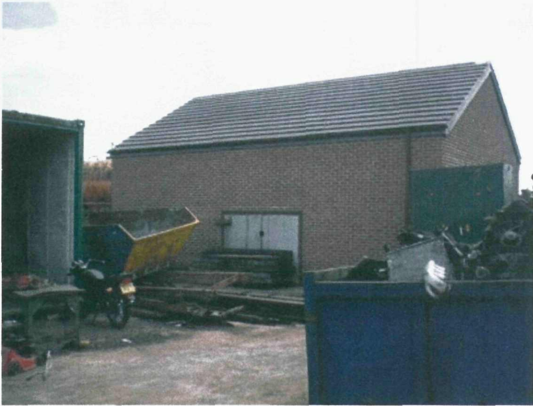
This is the second building identified on the plans to be demolished to make way for the proposed industrial unit.
