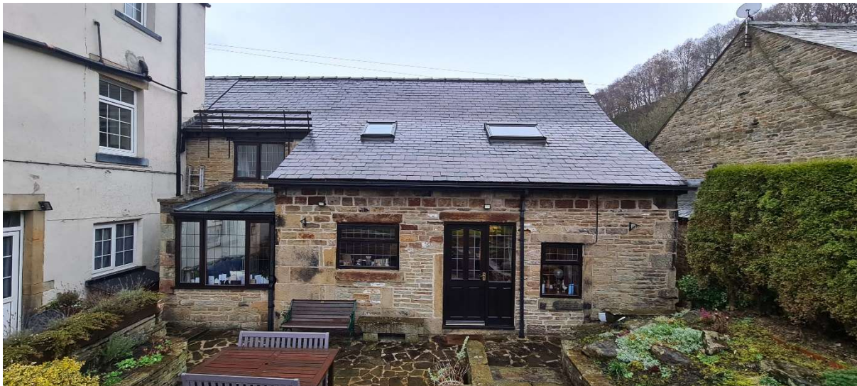
PHOTO 2: Rear elevation of Waterwheel cottage
