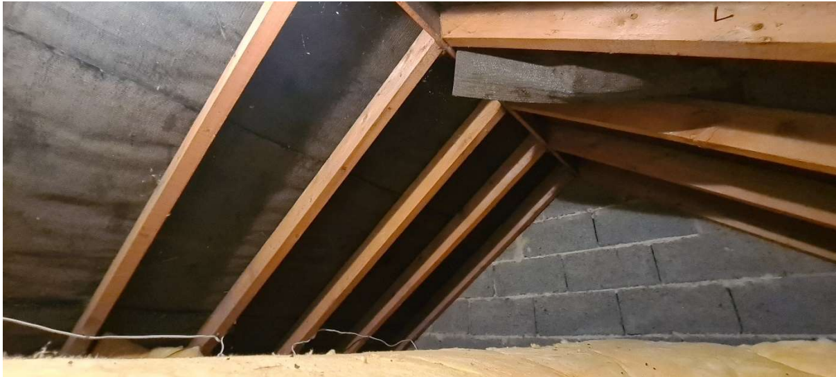
PHOTO 3: Roof void to be opened up & have conservation windows installed.
