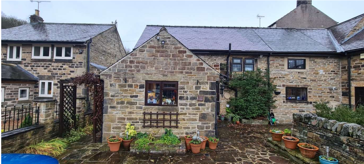
PHOTO 1 : Front Elevation of Waterwheel Cottage.
