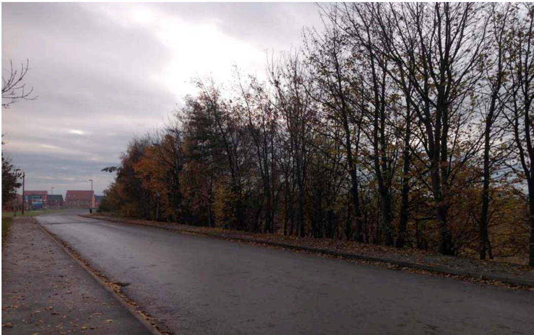
Figure 1- A view of G1 from the north.
