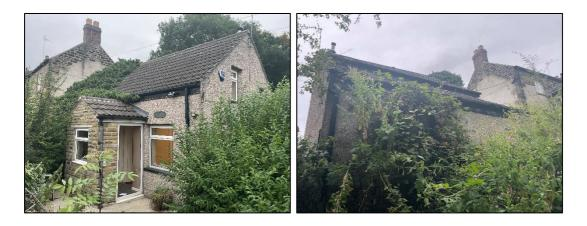
3.3.2. There is a small stone porch on the front of the cottage, also with a pitched roof covered with concrete interlocking tiles.
