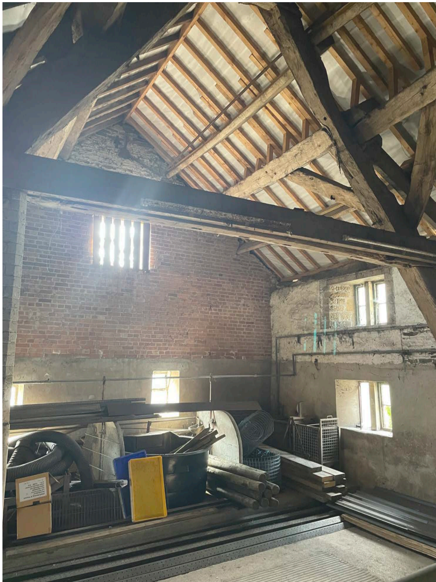
Photo Ref: E08 View of Nether Mill Barn (Internal Detailing Cruck Frame)
