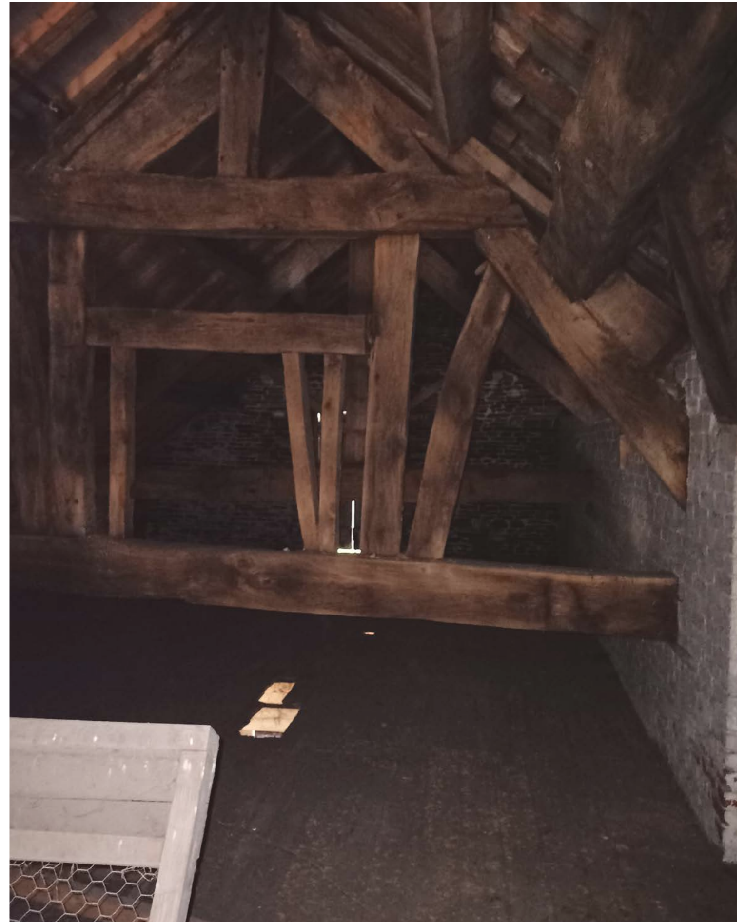
Roof Truss 4 Looking towards truss 5
