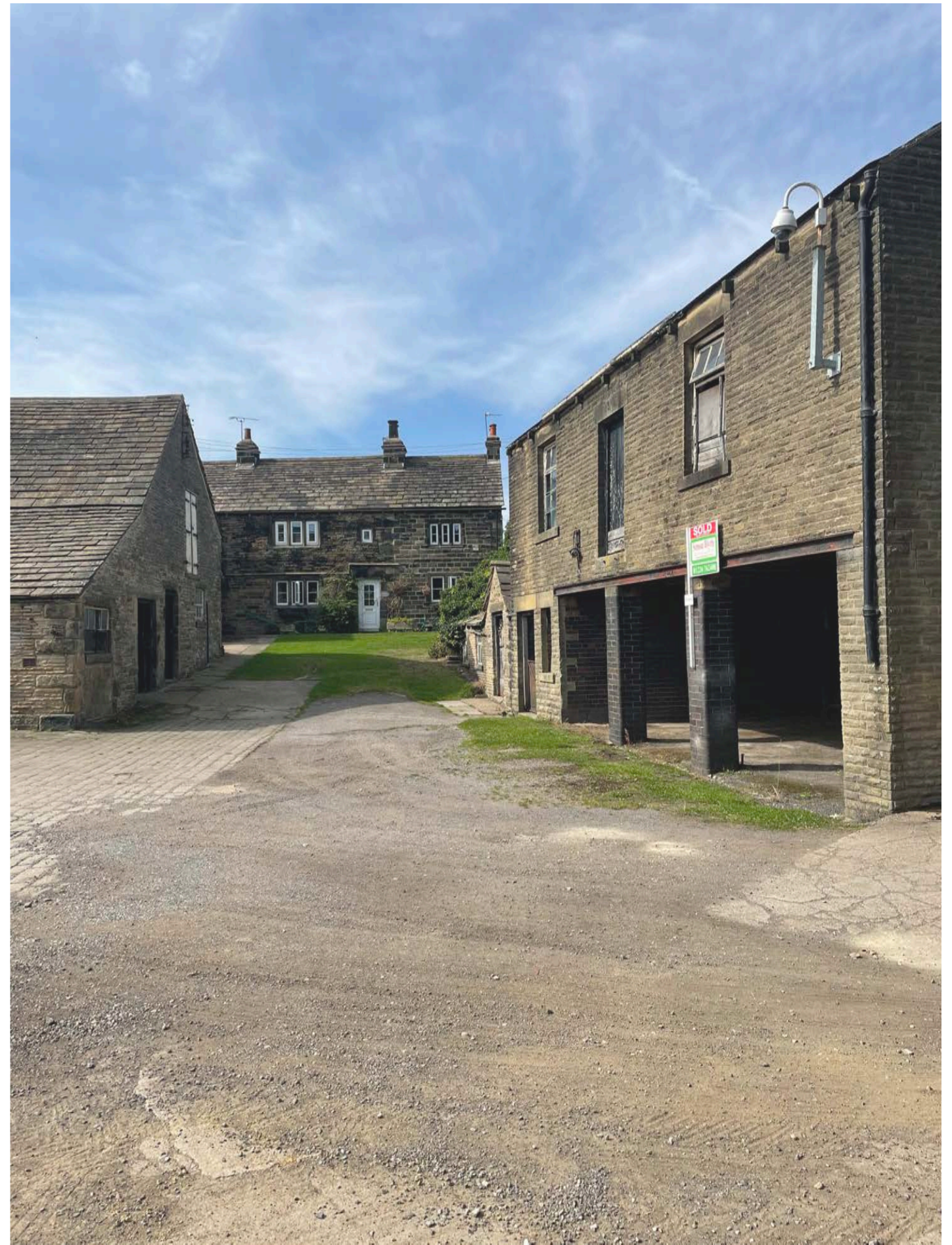
Photo Ref: E05 View of Nether Mill Barn (Side Elevation) from External Area
