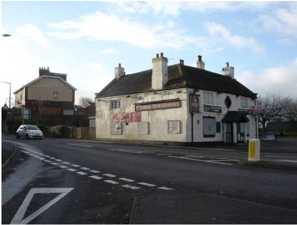
Fig 03. Public House from Jct with Church St
