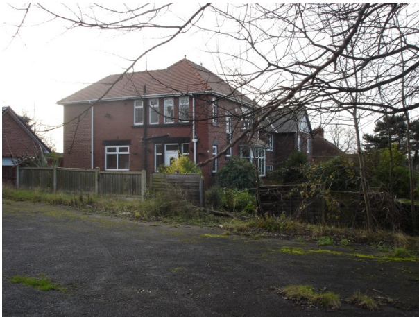
Fig 05. View of 5 Barnsley Rd looking west from site
