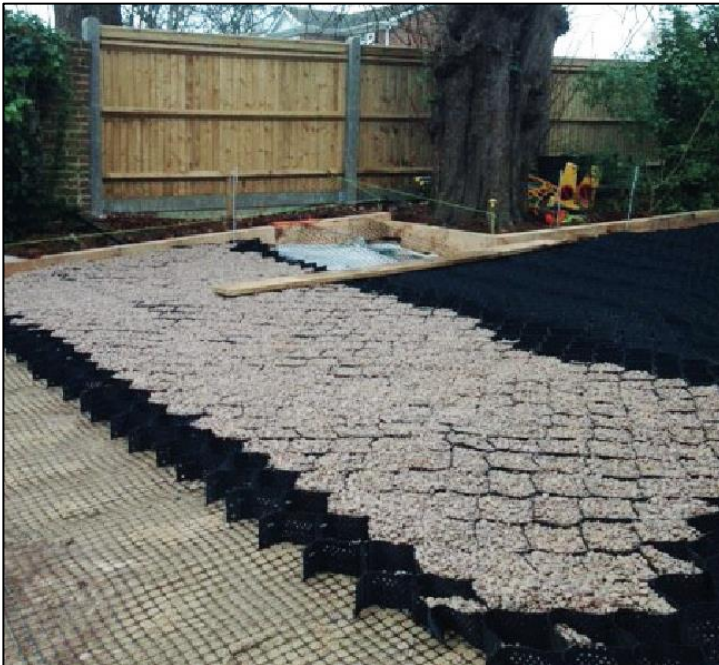
Figure A7.2: CORE TRP® geo-cellular confinement panels infilled with 4/20 mm clean, angular stone.
