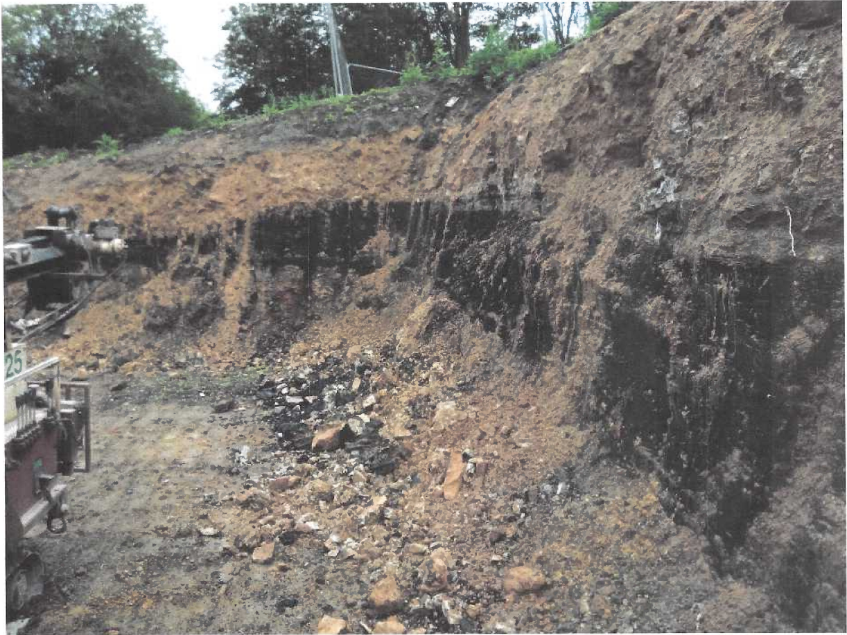
Exposure of probable Meltonfield Coal seam in excavation face
