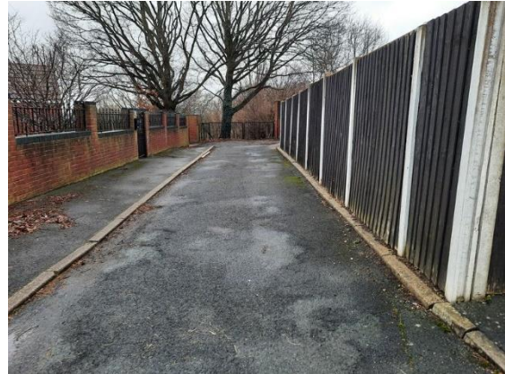
Plate 8.2: Hardstanding road within survey area
