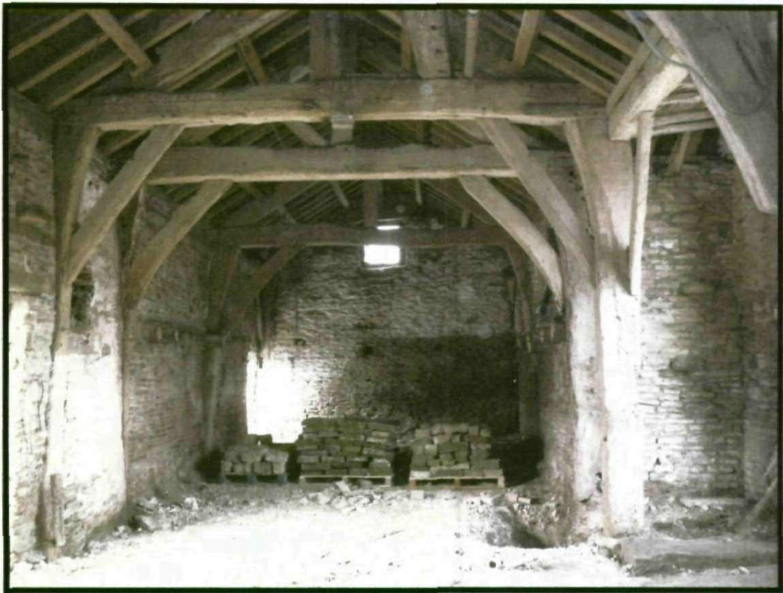
Photograph 10 – Internal view looking at North Elevation
