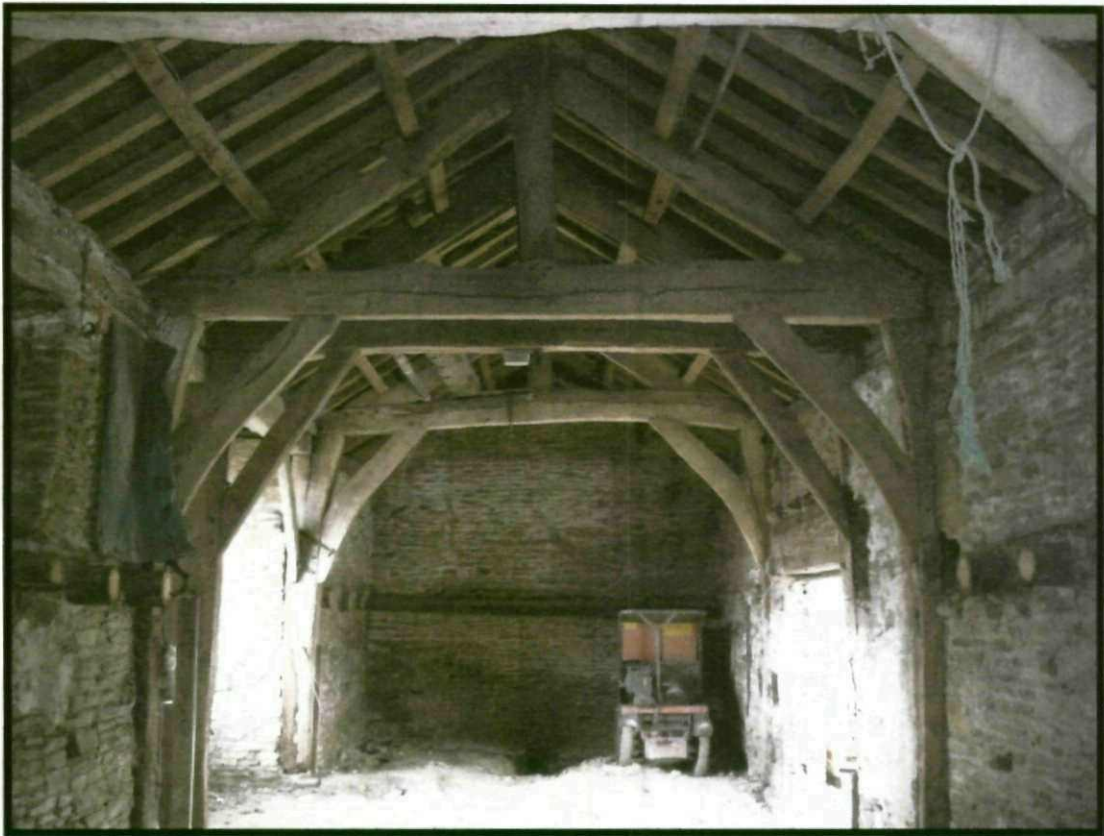
Photograph 12 – Internal view looking at South Elevation
