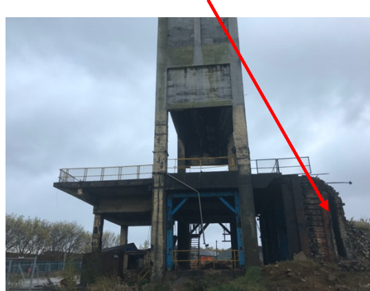
Image 26: Collapsed brickwork
