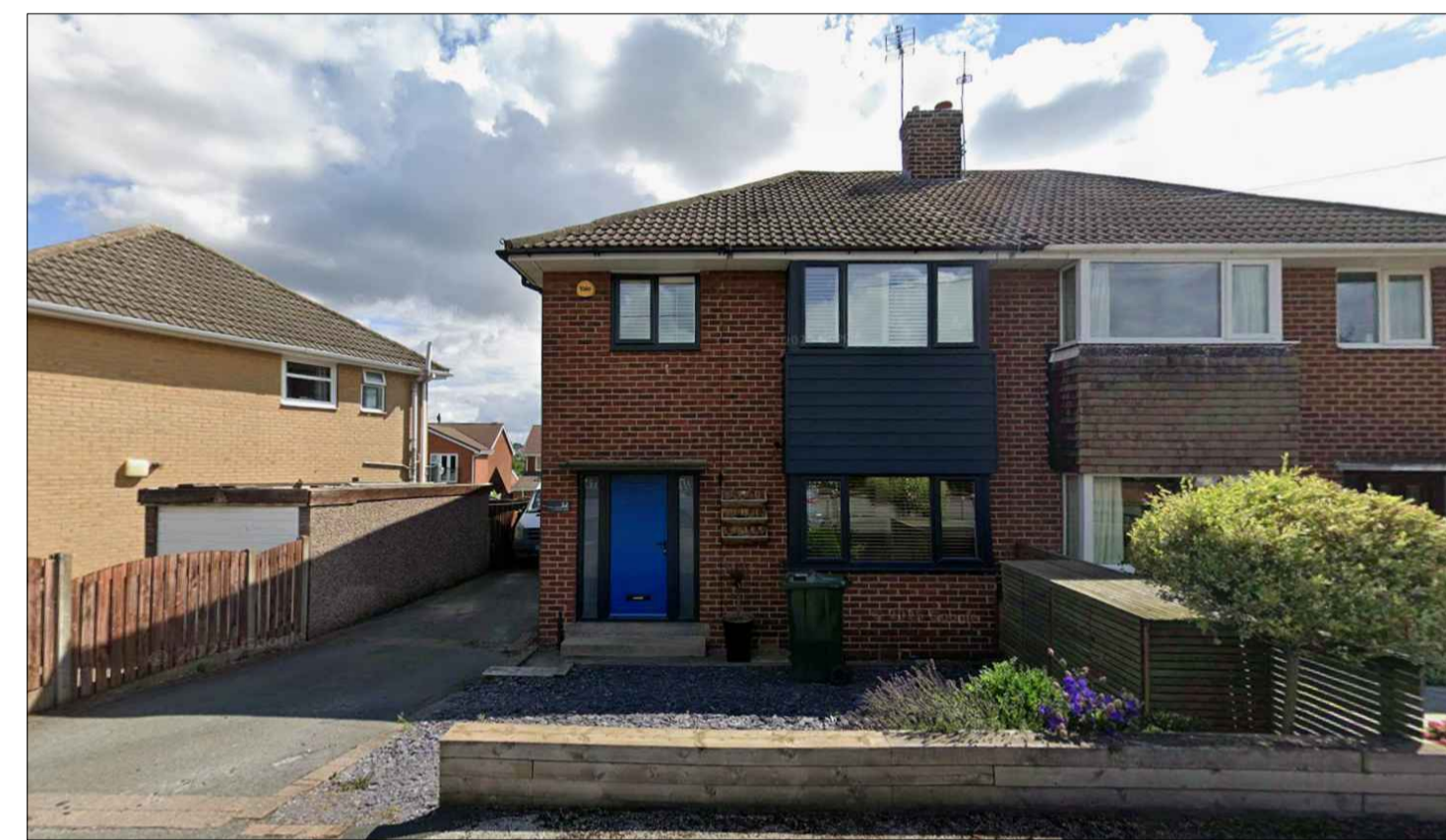
Photo of Existing Front
