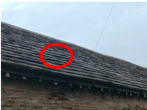
Photo 1: Bat emergence point on building (emergence survey 23/08/22).
