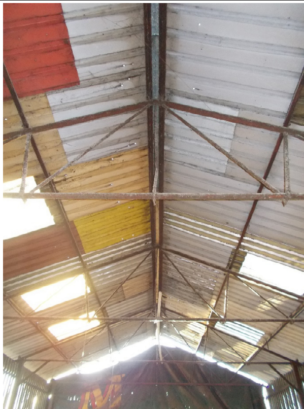
Photograph 4: Longitudinal view on steel roof structure
