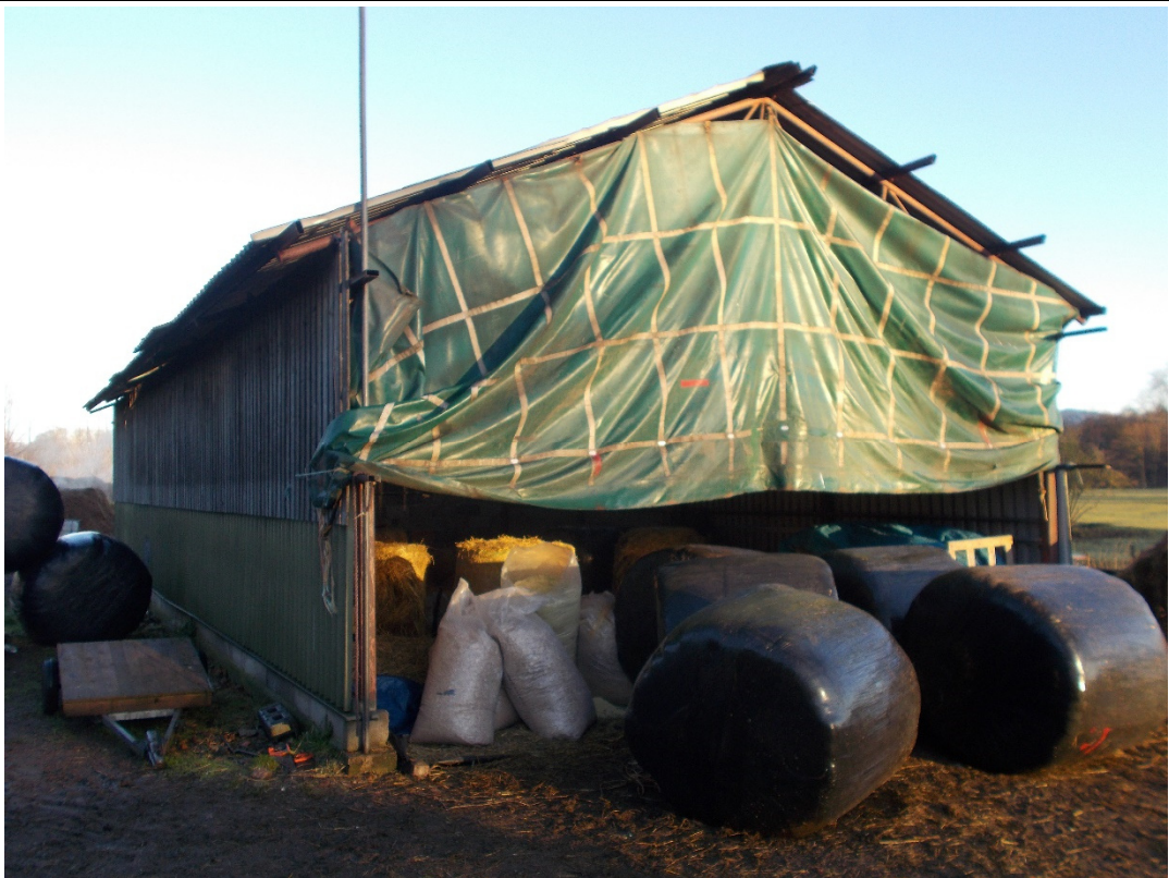
Photograph 2: External view from south west
