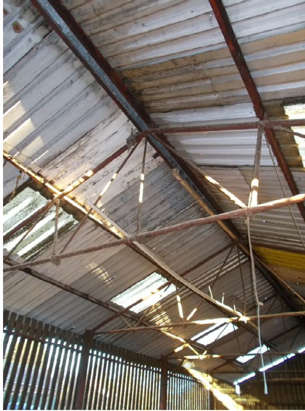
Photograph 3: Internal view on steel roof structure
