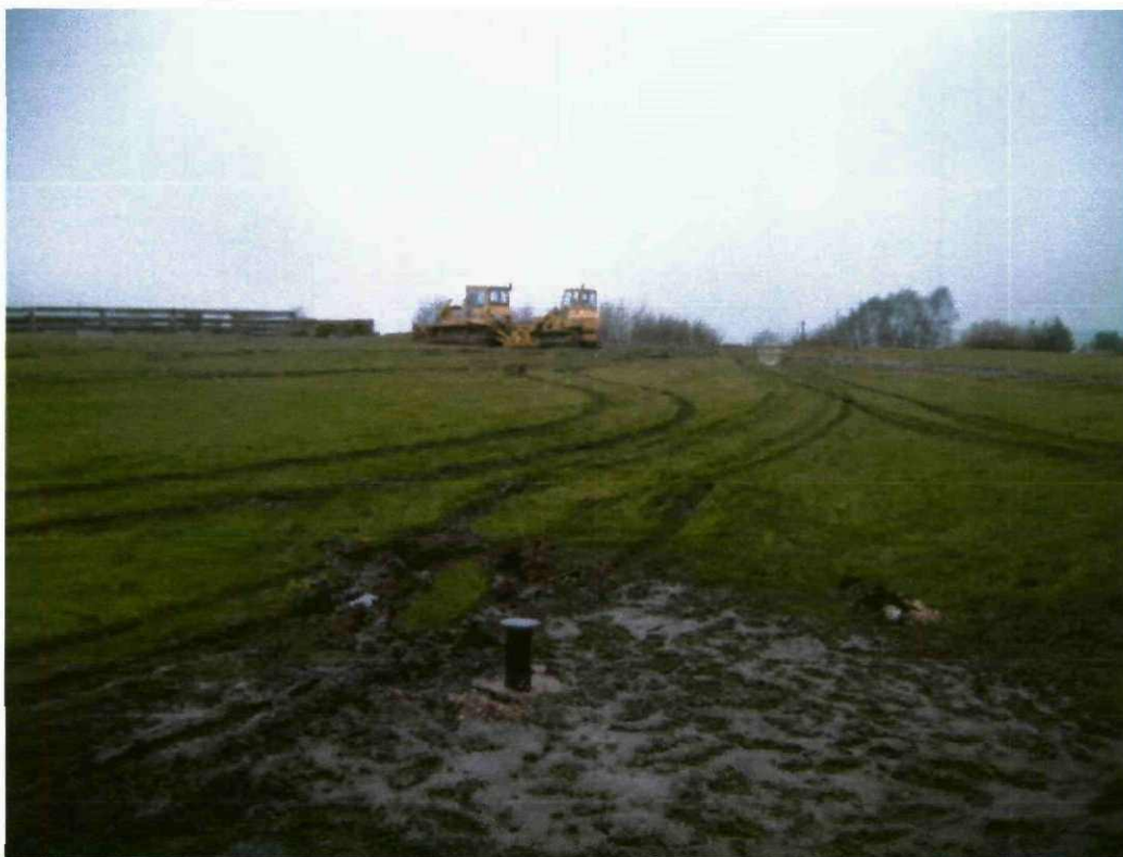
Photograph Number 13 showing borehole 9 drilled 25 th January 2011 for water and gas monitoring.
