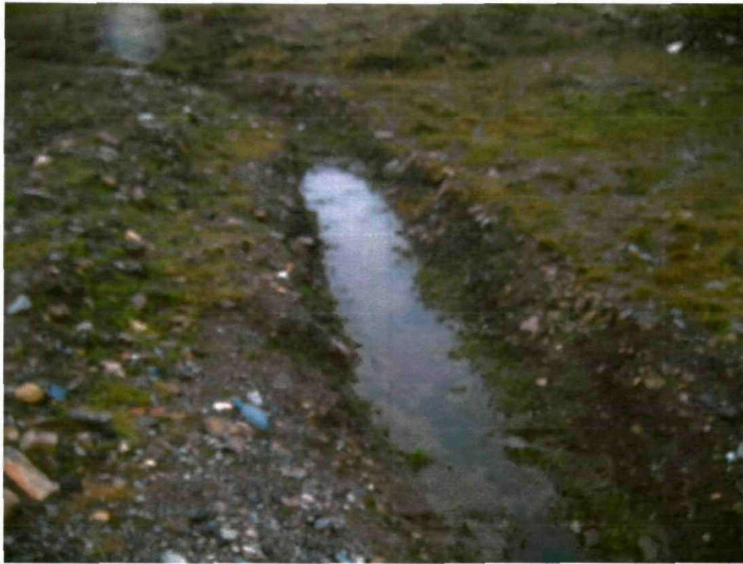
Photograph Number 7 showing the drain to the adit running across the site, monitoring point SW3.
