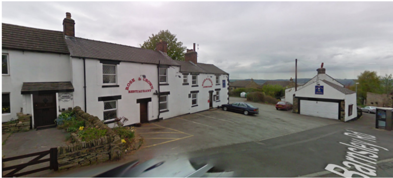
General View – Front Elevation from South
