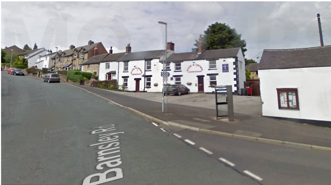
General View – Front Elevation from East (Barnsley Road)
