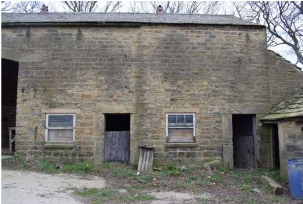
Fig 08. The cowhouse at the northern end of the barn with its two doors facing the yard
