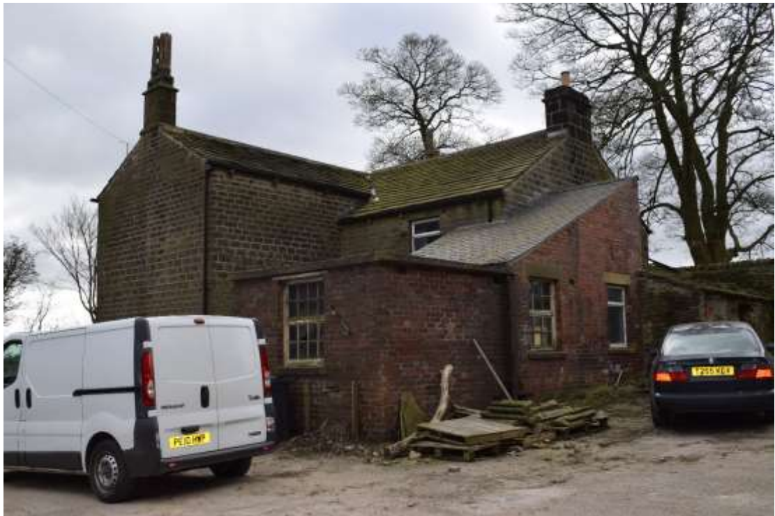
Fig 03. The rear of the farmhouse looking from the north-western corner of the farmyard
