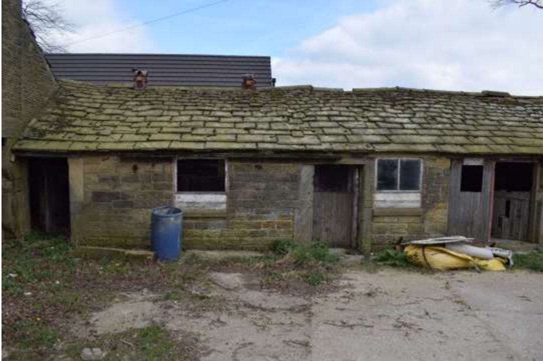
Fig 17. The western end of the cart shed range at the abutment with the barn
