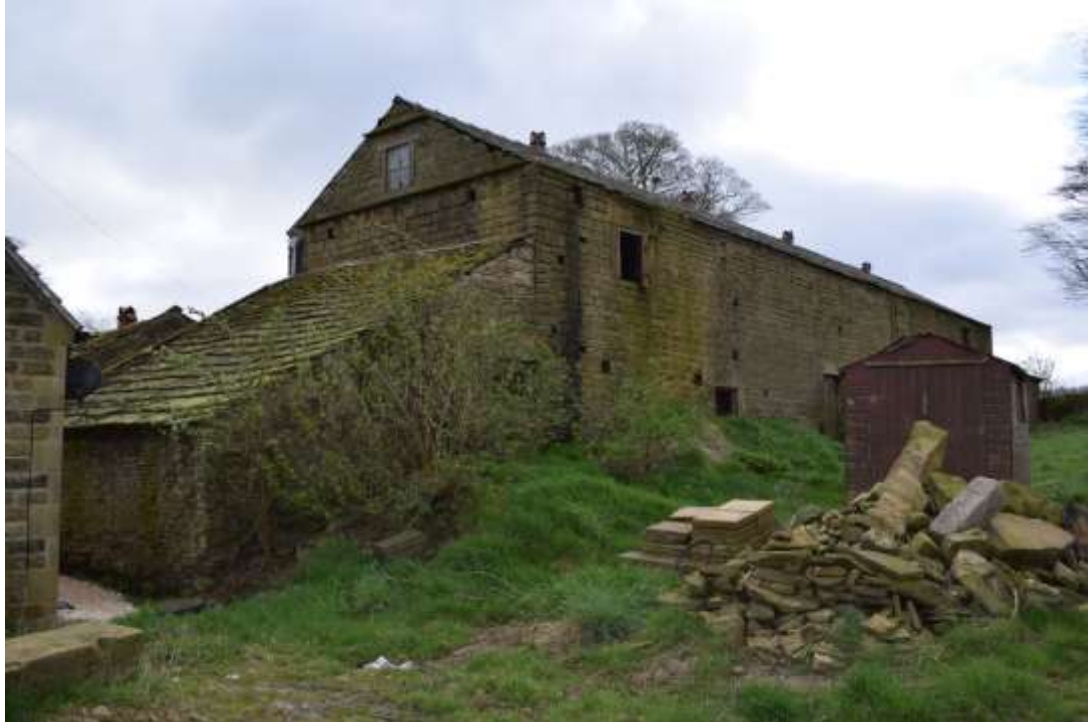
Fig 15. The lean-to link building at the junction between the combination barn and the cart shed range
