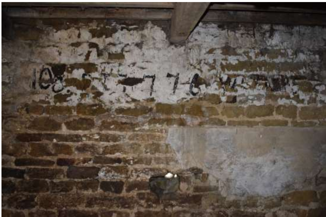
Fig 25. The internal face of the rear wall in the southern milking parlour (former oxen stable).
