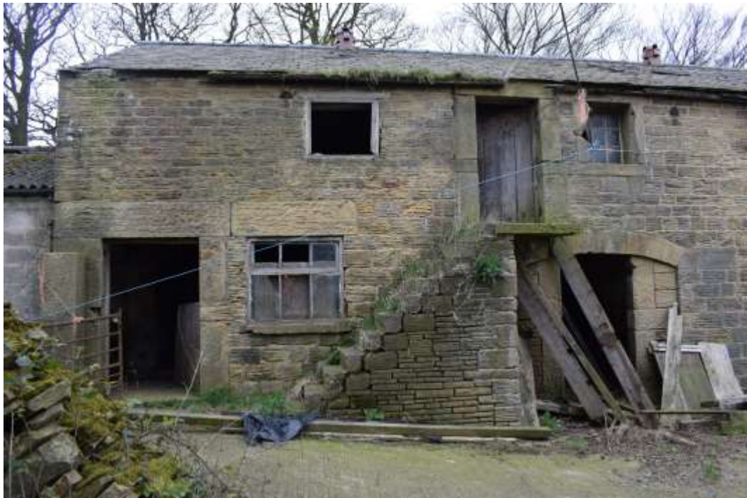
Fig 10. The southern end of the combination barn with the oxen stable, external stone staircase to a hay loft and the partially blocked small cart opening
