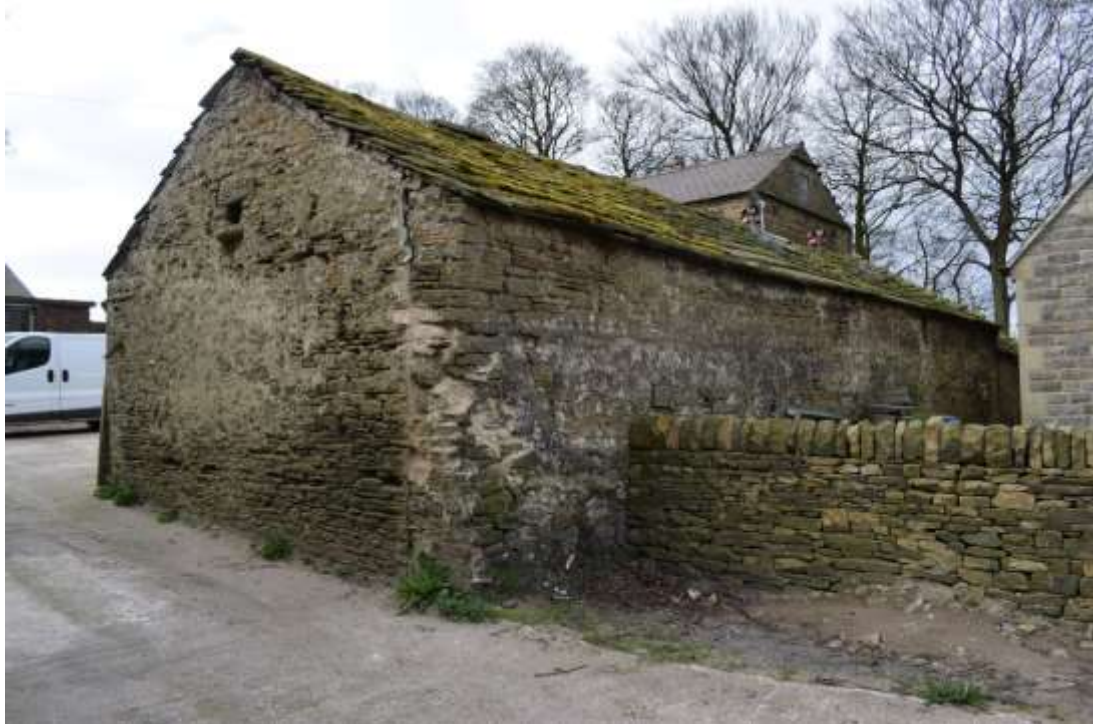
Fig 28. The north-eastern corner of the cart shed range from the north which frames the only vehicular access into the farm yard.
