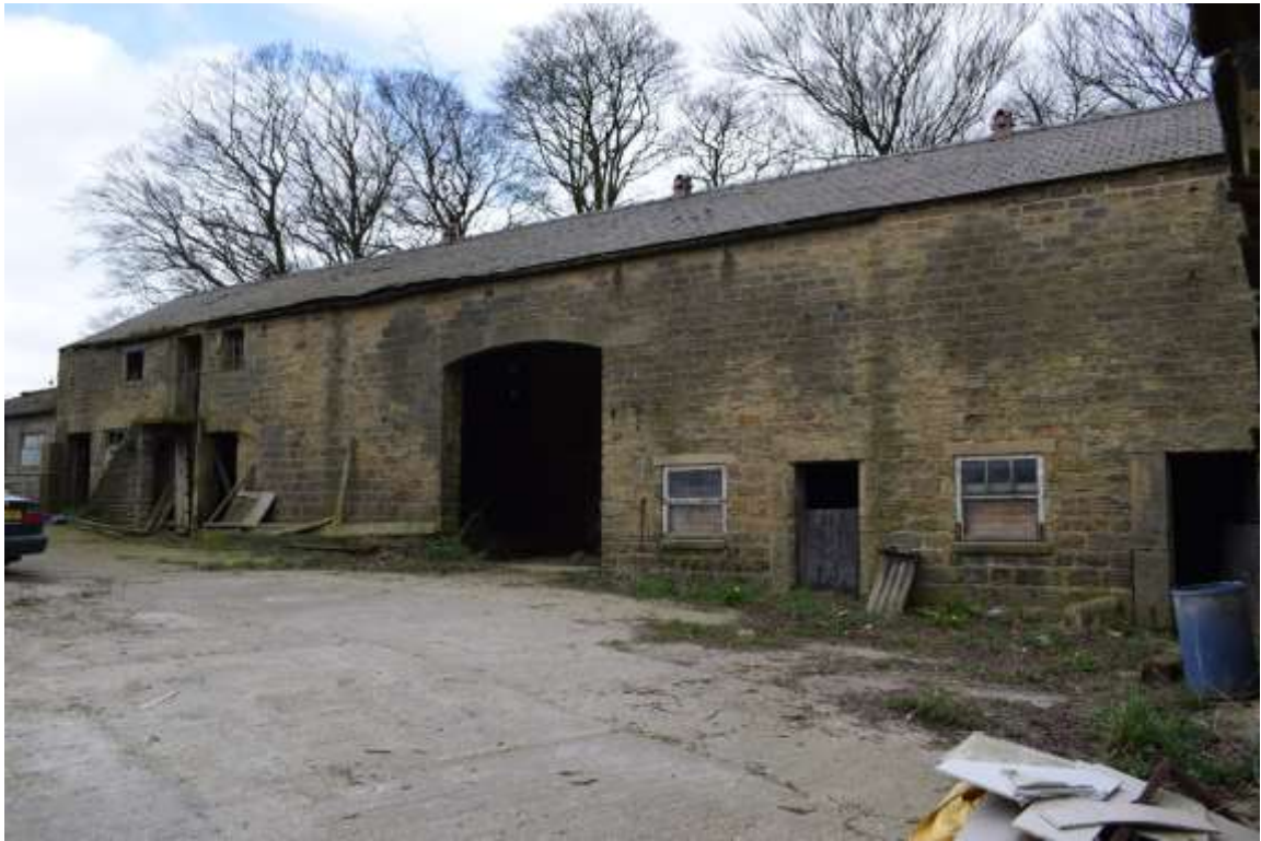
Fig 01. Front elevation of The Barn, Cliffe House Farm
