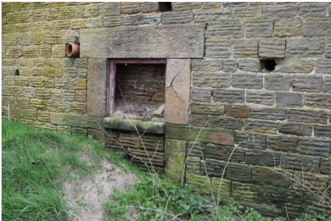
Fig 09. The opposing cowhouse door in the rear of the barn
