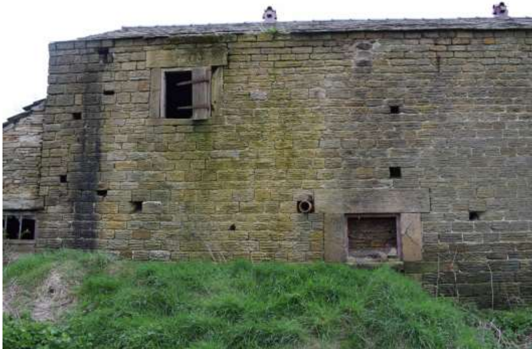
Fig 12. The pitching eye at the northern end of the rear (western) elevation
