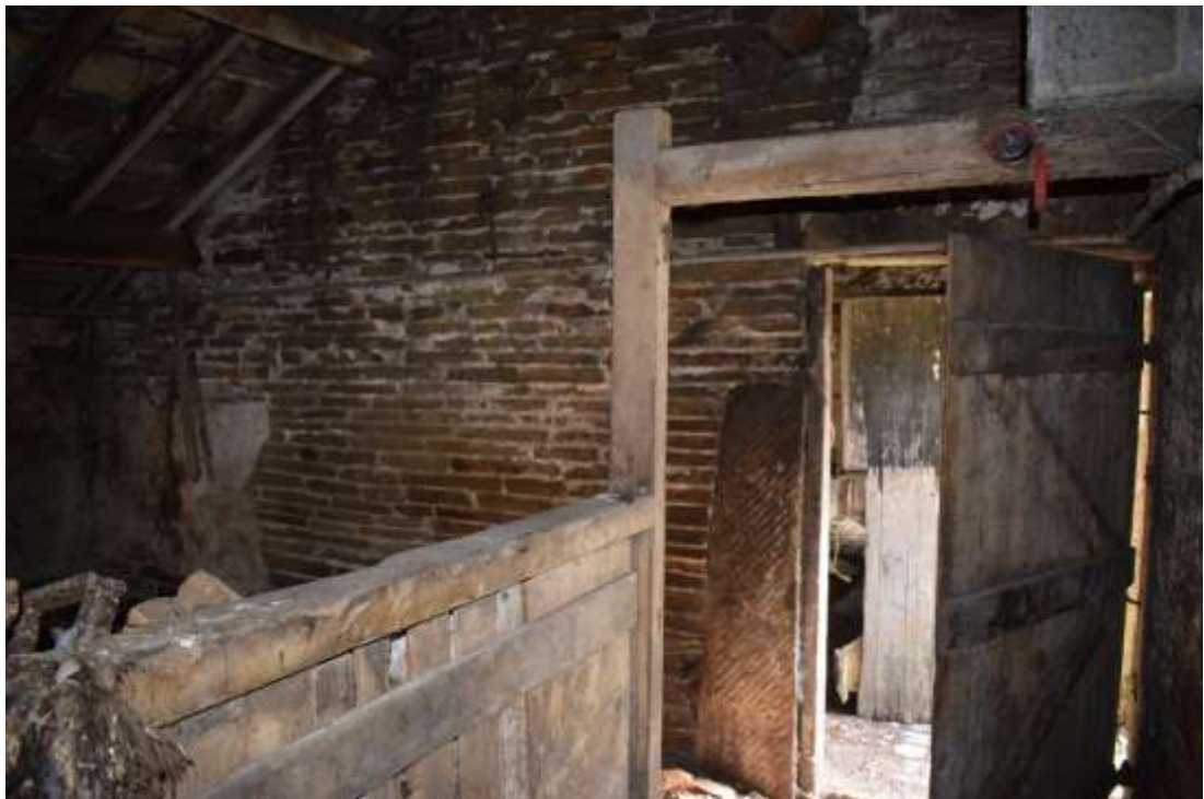
Fig 27. The interior of the link building showing the stall enclosures (looking east towards the cart shed range) and a gate post forming the jamb of the door into the cart shed range.
