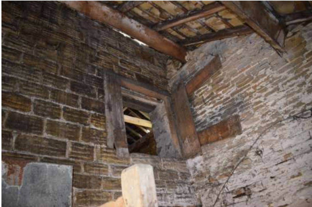
Fig 26. The internal junction between the barn north gable and the link building (note the low level pitching eye from the northern hay loft in the barn).
