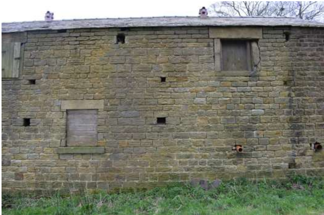
Fig 13. The pitching eyes at the southern end of the rear (western) elevation and the later ground floor window which lights a corridor behind the cart store
