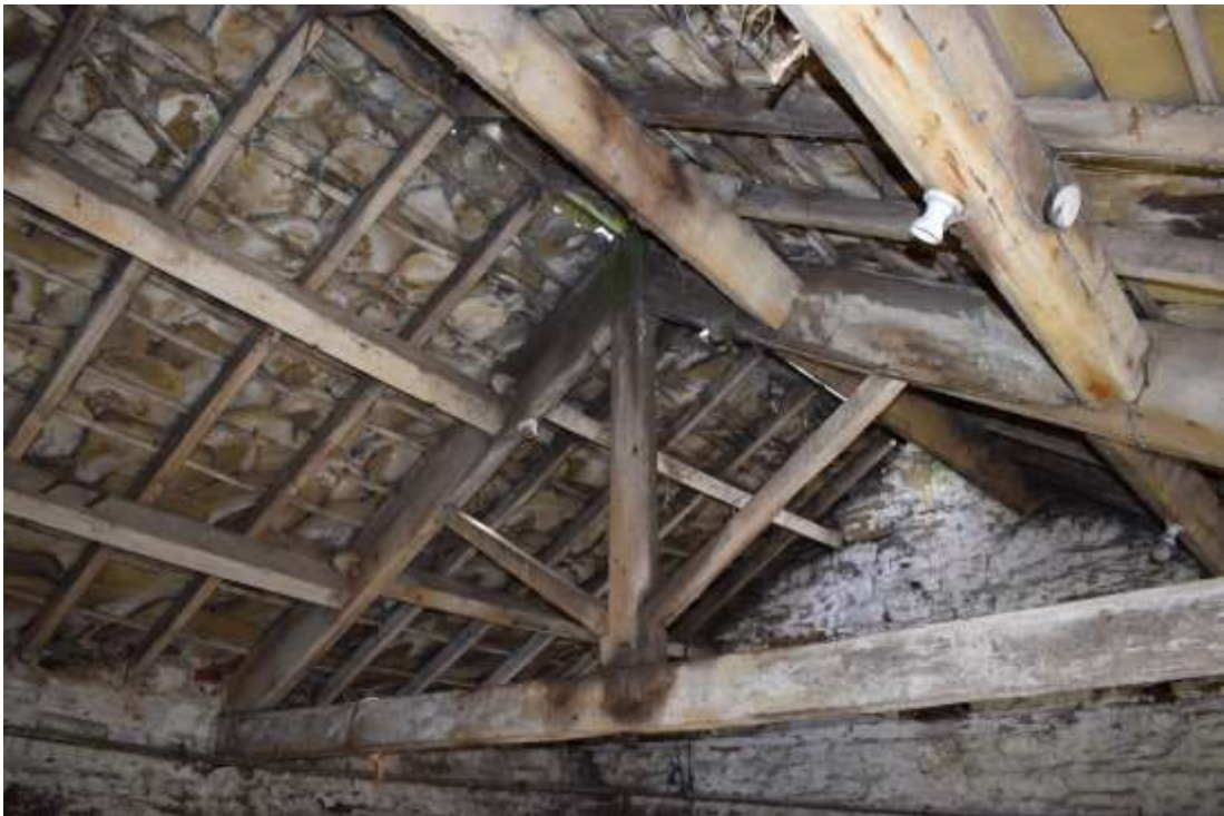
Fig 18. The cart shed roof structure (looking east)
