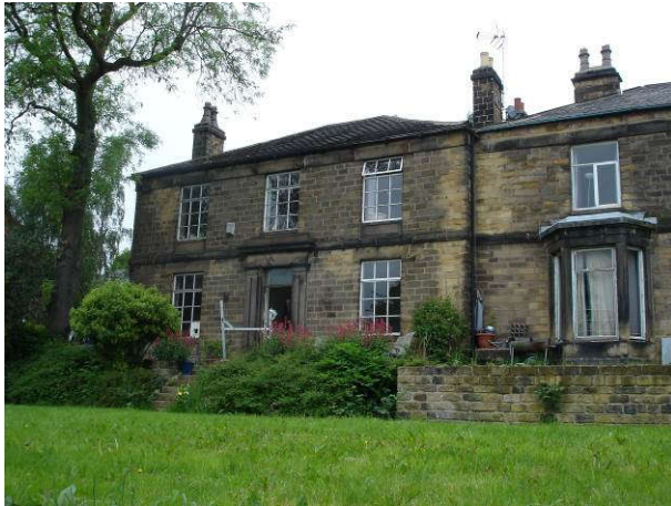
Fig 04. Darley House to the north
