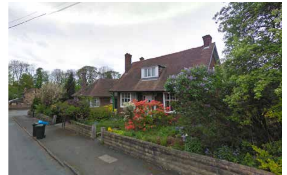
View of the site along Tivy Dale Close
