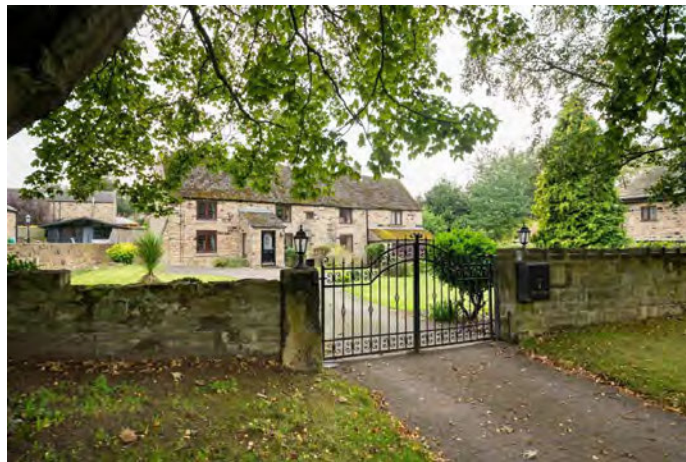
View Of Hirst Cottage From Chapel Lane
