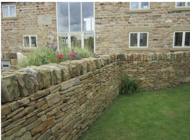
Dry Stone walling on the development
