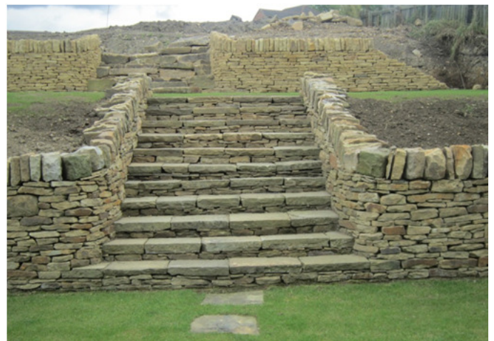
Dry Stone walling on the development
