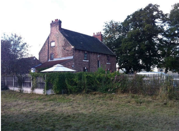
Fig 05. Rear view of Hall Farmhouse from rear garden of the building plot looking south west.
