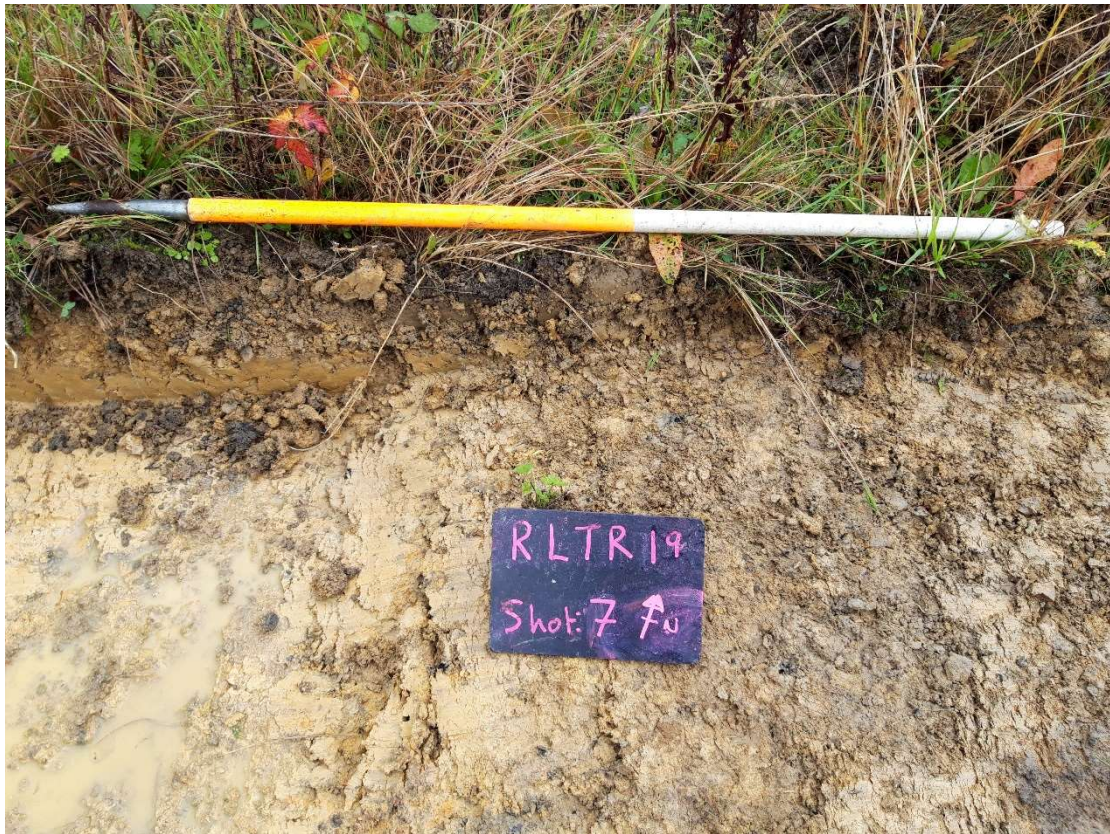
Plate 5: Section 4, looking north (damage A)
