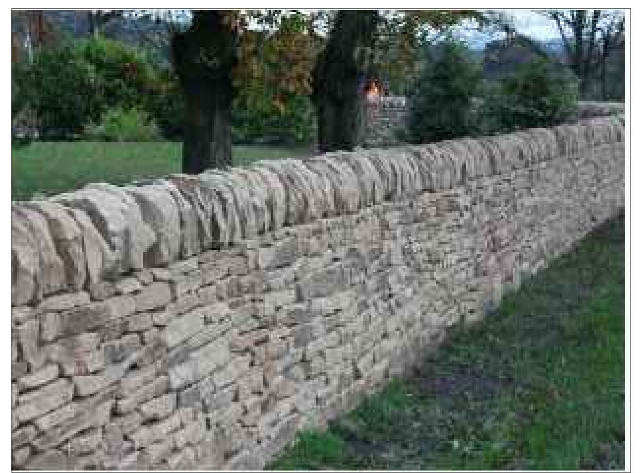
Dry stone walling feature to entrance bellmouths. (behind Visibility Splays) approx 1500 high min 25m length (each) built using local / reclaimed stone by a Local Stonemason
