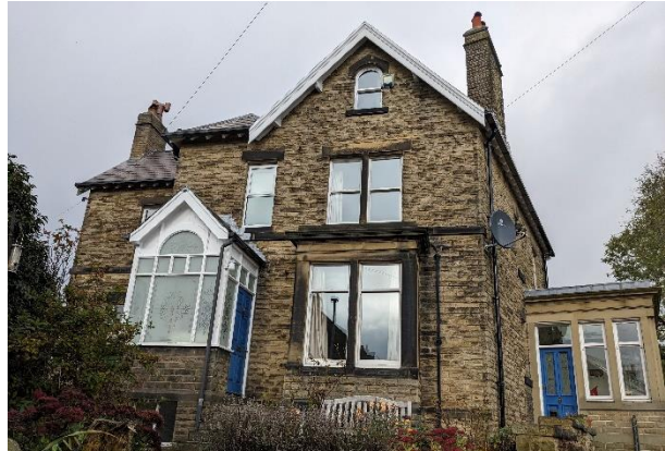
Existing South elevation of 103 High Street
