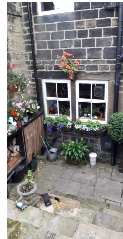
Existing windows to be left uncovered due to extension
