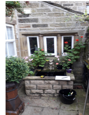
Stone ashlar lintol/sill and mullions to be reused in new extension
