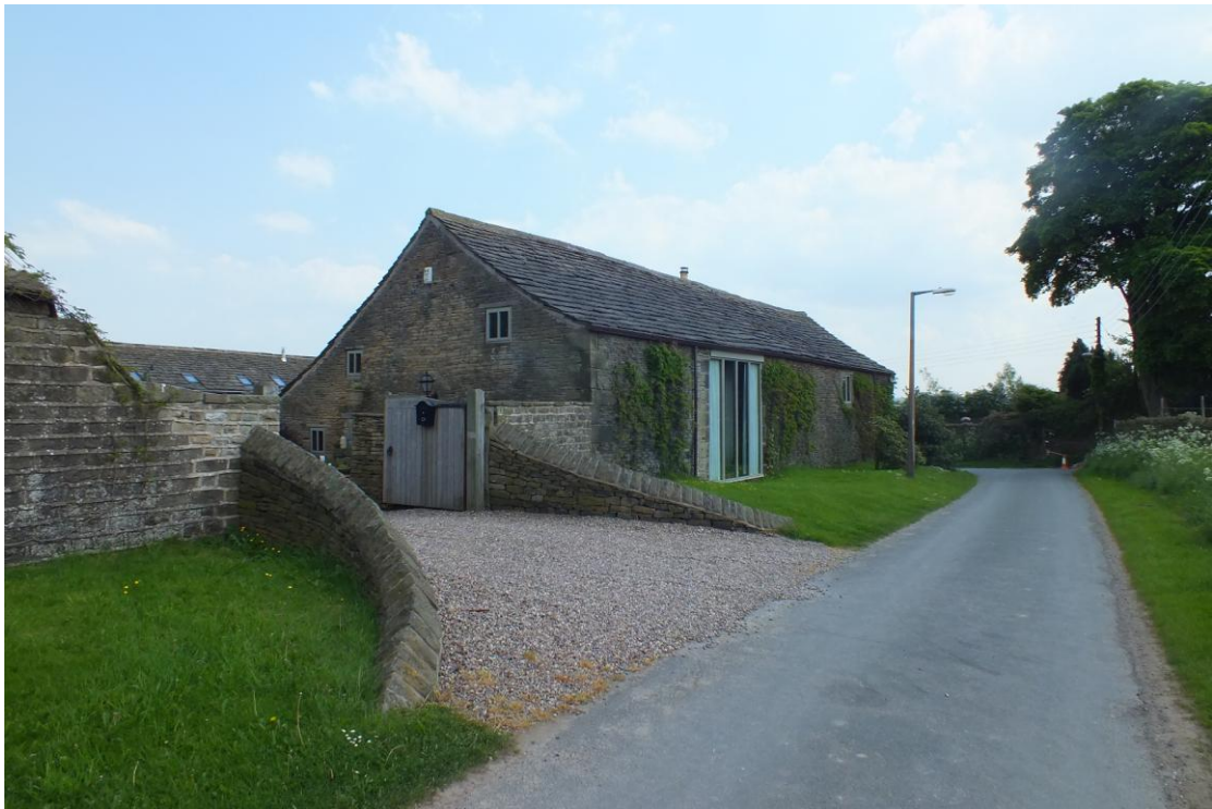
Image 4.11 - View from west of Conservation Area and Gr II* listed barn
