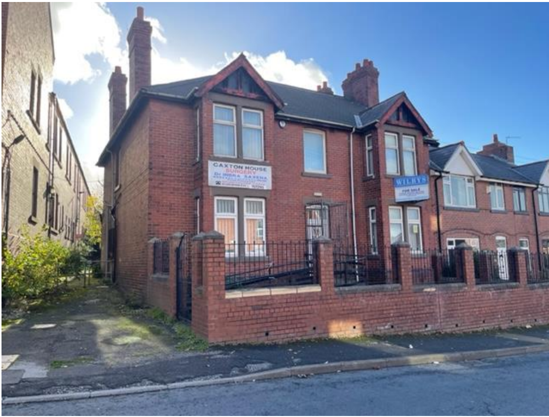
Front elevation of the building.
