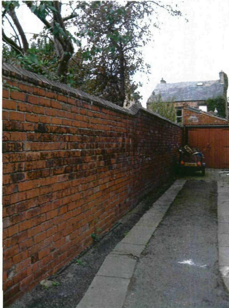
5. Existing high brick boundary walls enclosing the site.
