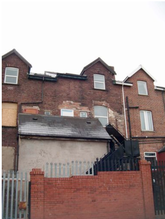
Figure 3 – View of rear elevation no. 47
