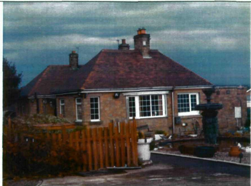
Photograph 7 – Above is the existing property which is on site, which is proposed for demolition once redevelopment takes place.
