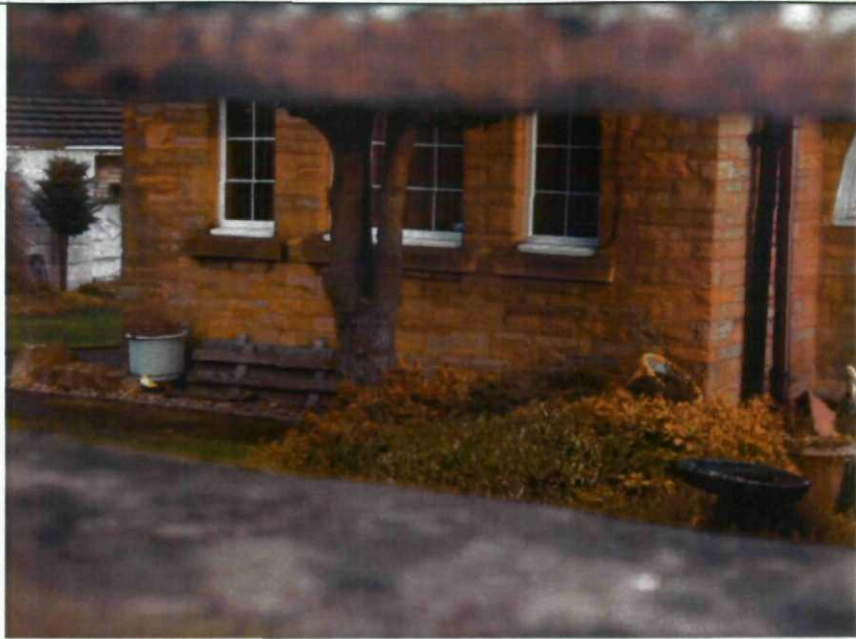
Photograph 9 – The above shows the side elevation and landscaped gardens on site.
