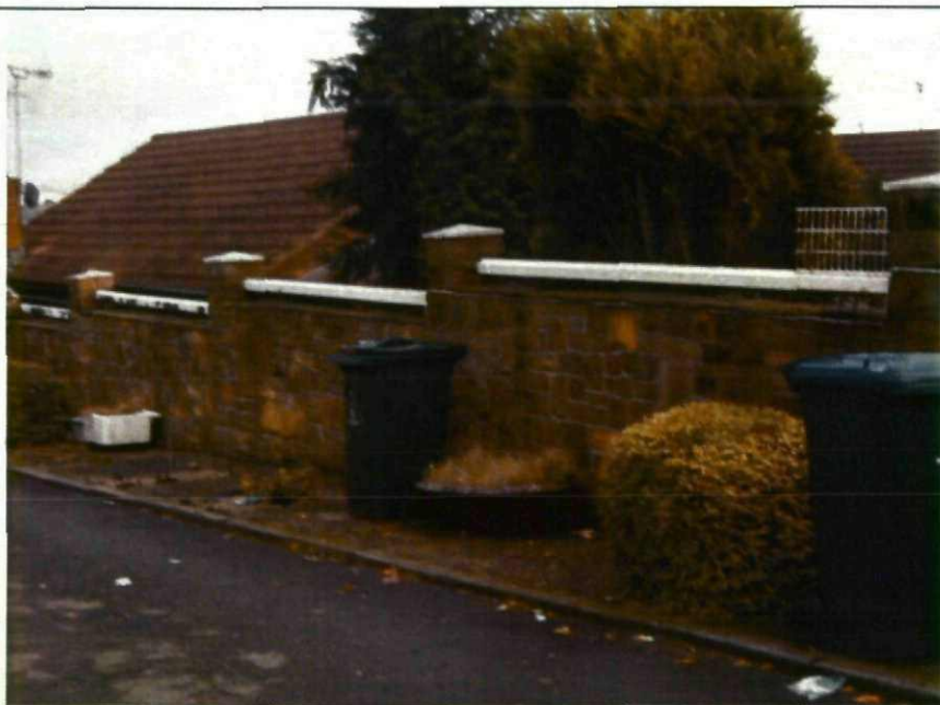
Photograph 4 – The boundary wall to the right hand side of the entrance upon entering the site.
