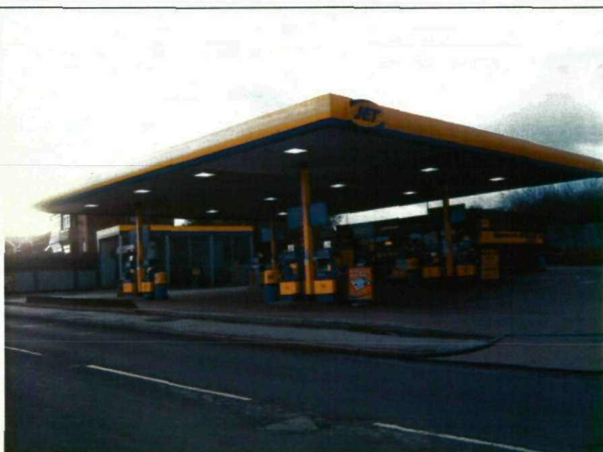
Photograph 12 – The above shows a fuel station adjacent to the existing site located on Burton Road.
