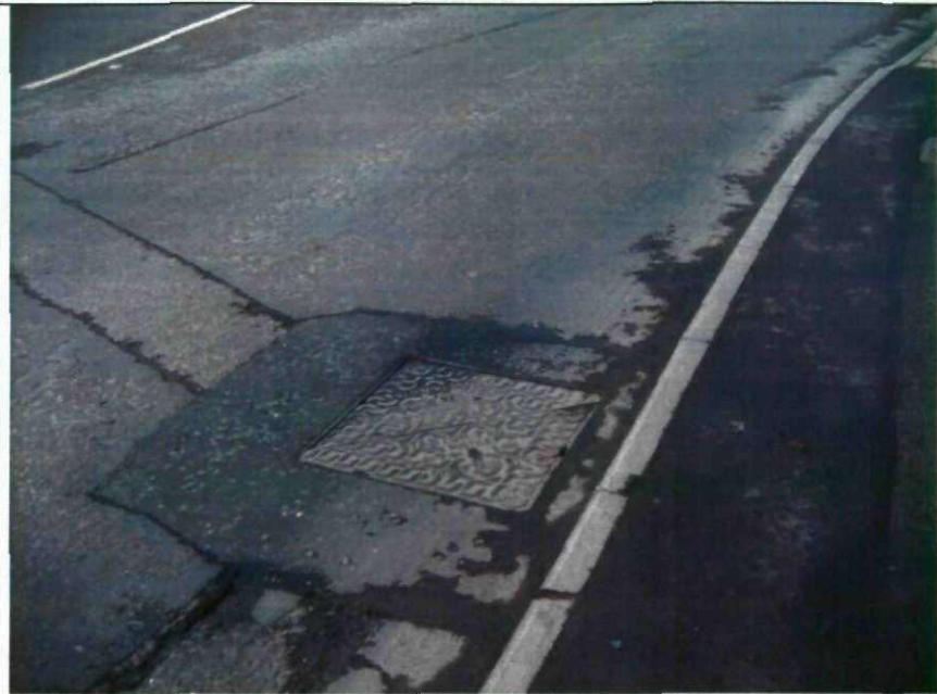
Photograph 13 – Outside the north west boundary of the site on Burton Road was a manhole.
