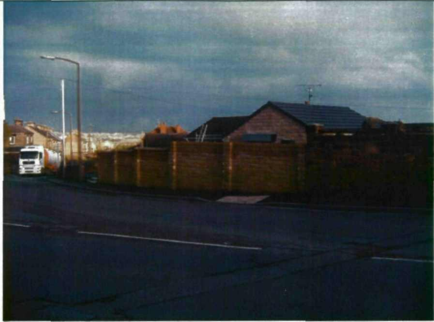
Photograph 1 – The above shows Burton Road in the foreground and part of the boundary wall to the existing property.
