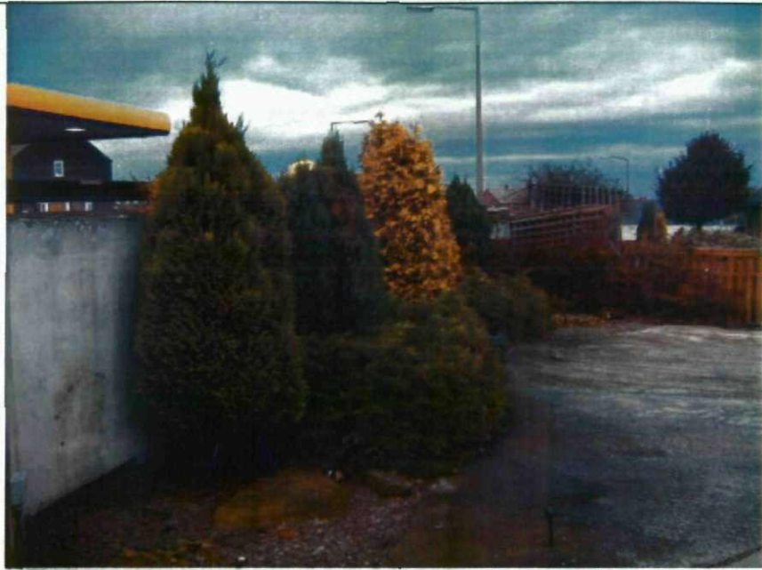
Photograph 5 – The boundary wall to the left hand side of the entrance upon entering the site.
