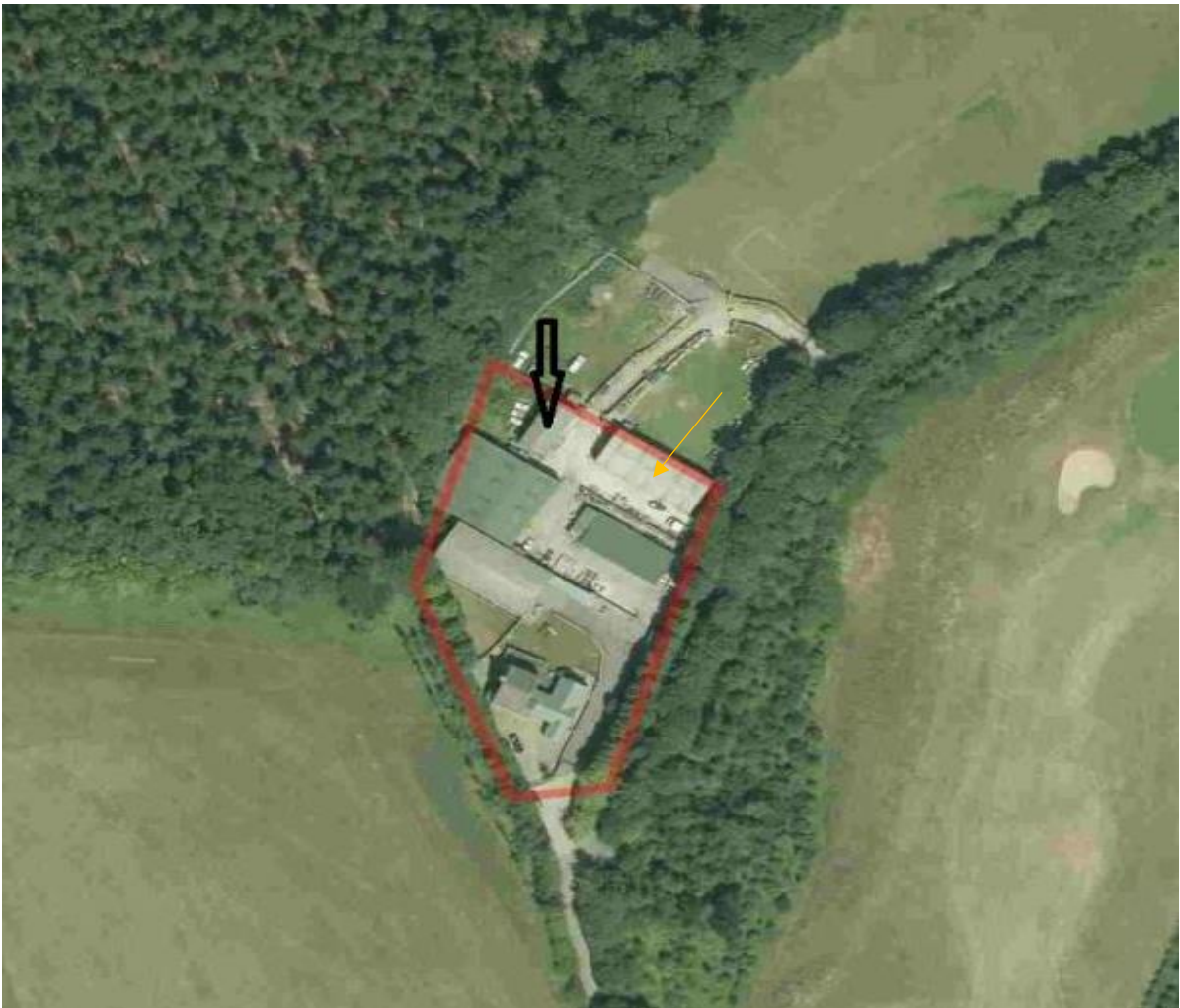
Fig 1 - Aerial photograph: Annexe Barn (shown with black arrow) - Anchor Farm, Elmhirst Lane, Dodworth, South Yorkshire, S75 4LD
