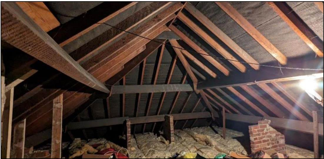
Plate 8. Building 1 roof void
