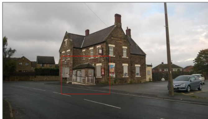
Pic 4: Access ramp and entrance to be demolished
