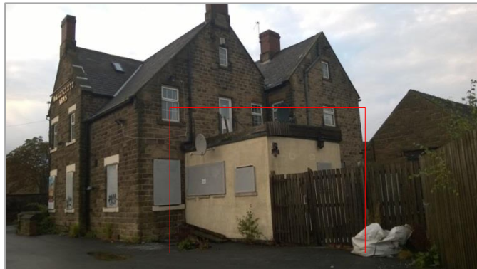
Pic 3: Extension to be demolished
