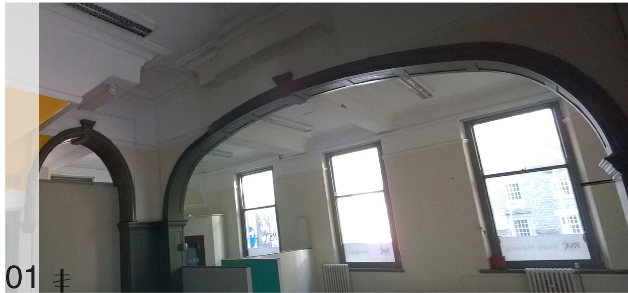
Arch features in main office space
