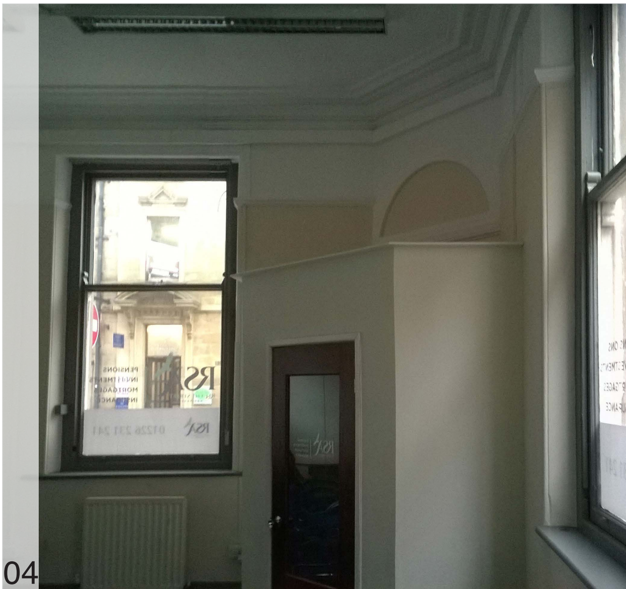
Plaster coving and features in main office space
