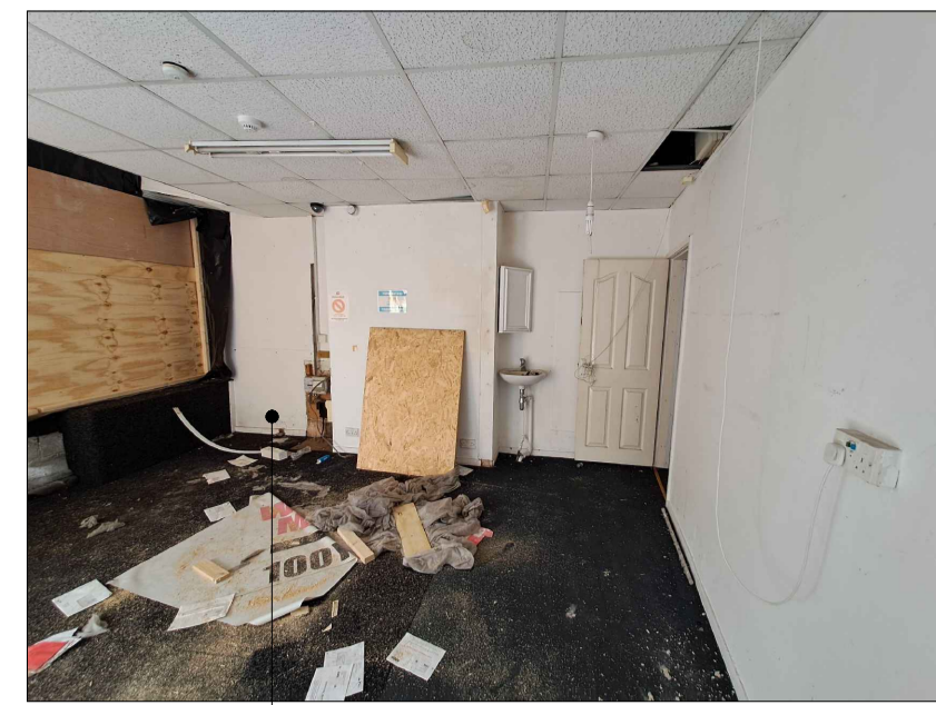
Indication of finishes in No.307 (vacant retail) ground floor accommodation
