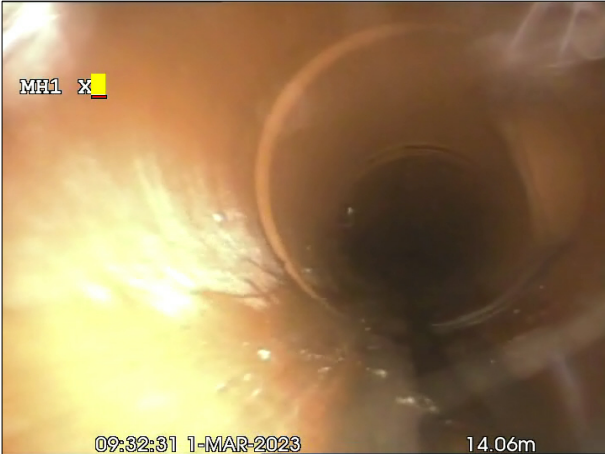
Photo: 16_8a, 00:00:00 14.1m, Junction at 03 o'clock, dia 100 mm
