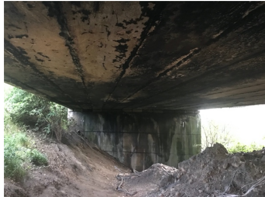
Image 2: Underside of bridge deck
