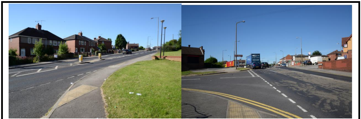
View along and to the Rotherham Road/Pontefract Road junction showing pedestrian refuges and dropped crossings.
