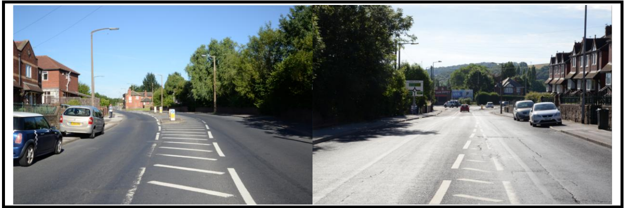
View north and south along Rotherham Road
