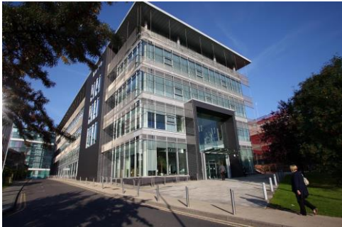
Barnsley Metropolitan Borough Council (Westgate Plaza One)
