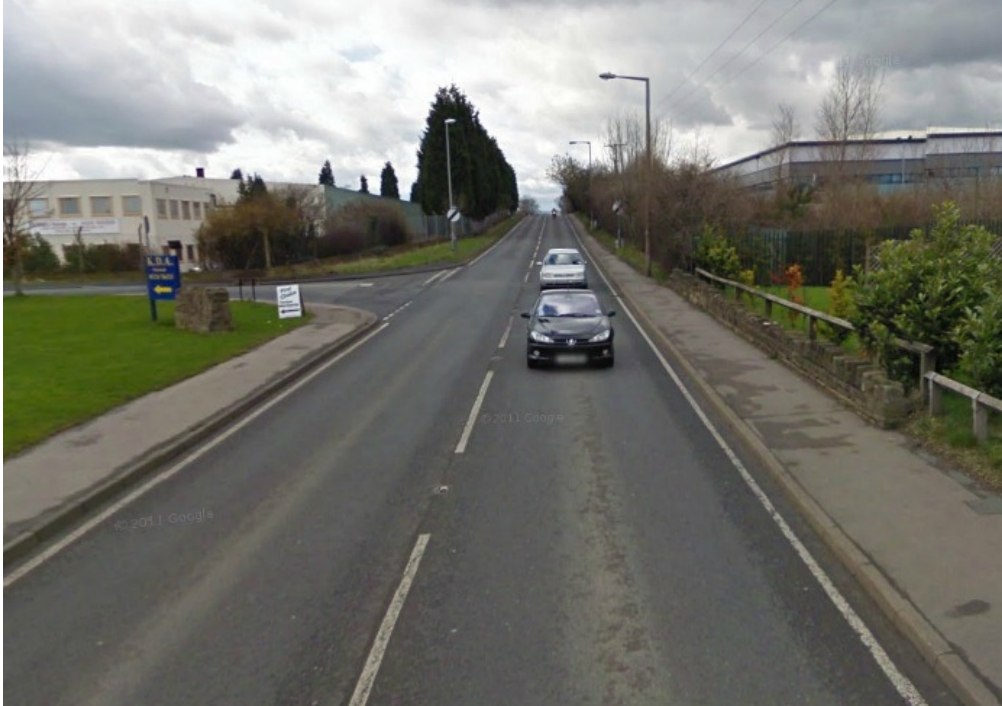
Photo 3 – Barnsley Road, A628
