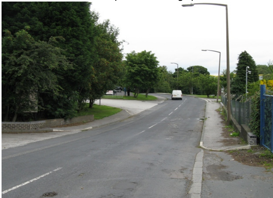
Photo 1 – Fall Bank Crescent (site access on right)
