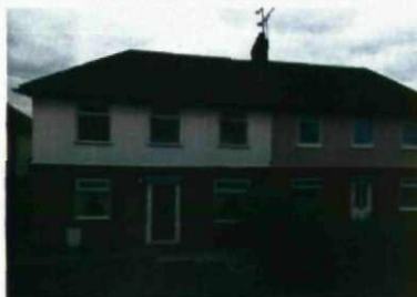
Typical Hawthorne Crescent semi-detached property
