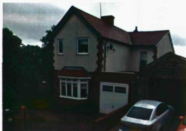
A more modern Barnsley Road property
