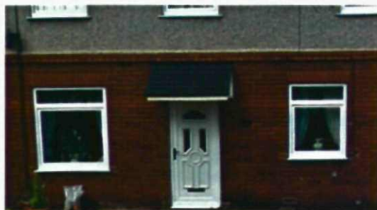
Architectural detailing along Higham Lane
