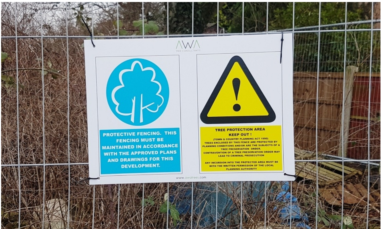
Figure 5: Example of A3 tree protection warning sign fixed to fencing panel
