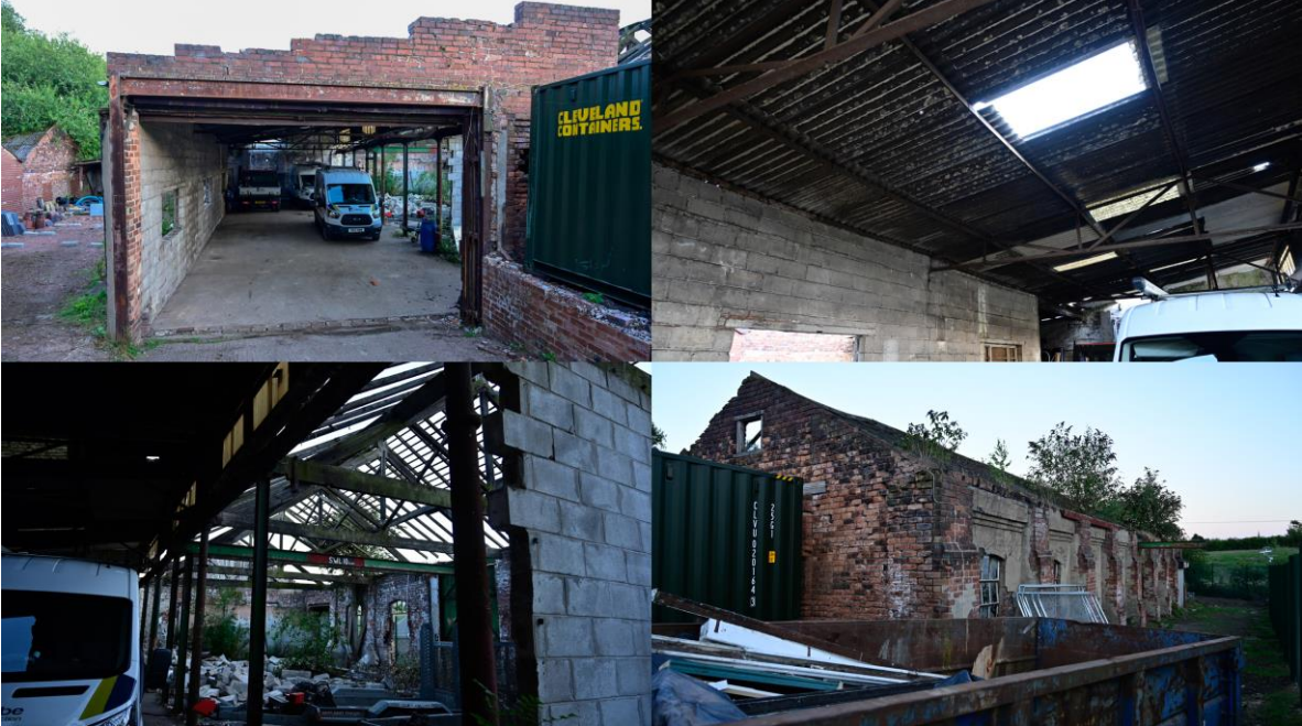
Photo 2: Various aspects of building 2
