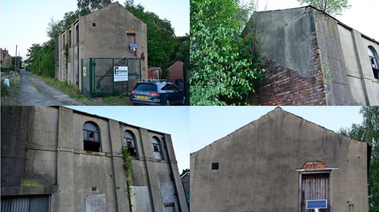
Photo 1 Various aspects of building 1
