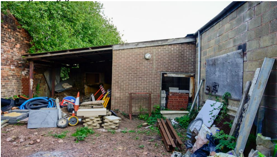
Photo 4 Lean to shed identified as building 4
