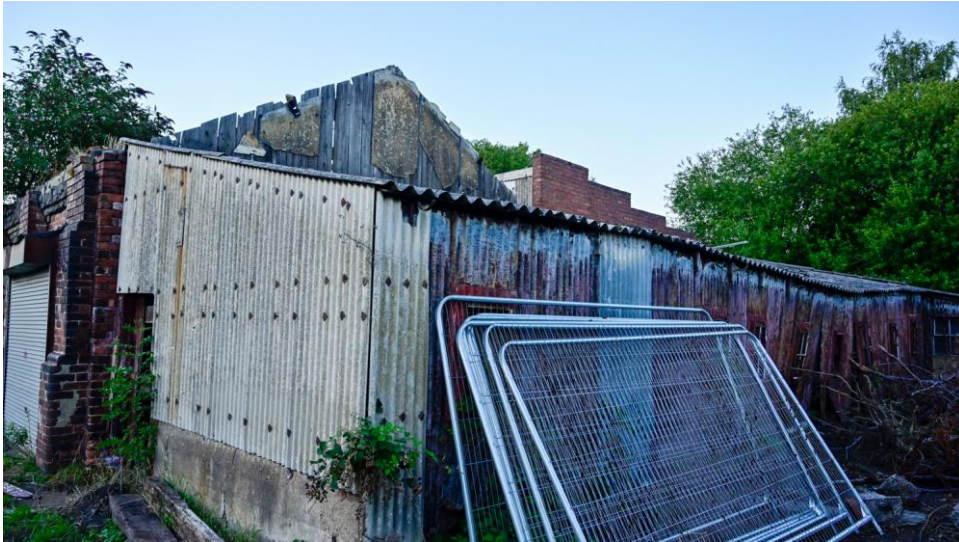
Photo 3. Building 3 at south end of the site
