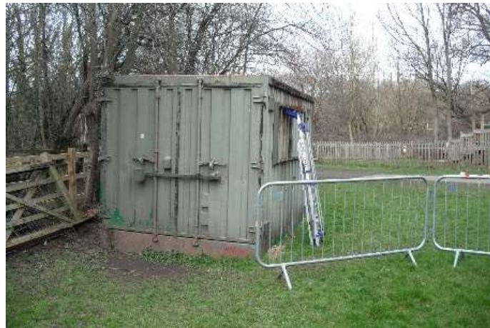
Existing Container placed near the hedge and public footpath
