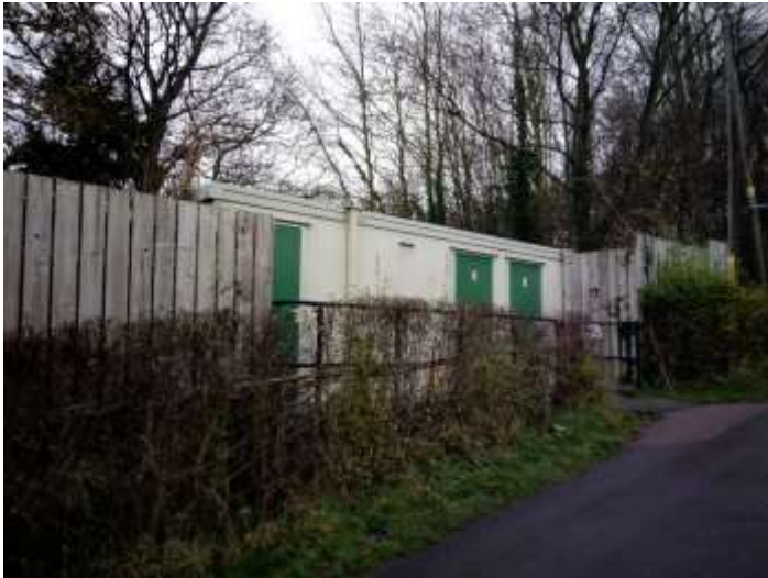
Existing toilet block
