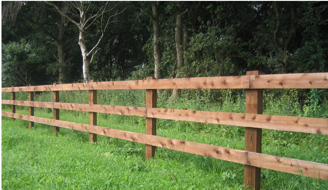
Figure 1 Typical timber fence to restrict access to trees
